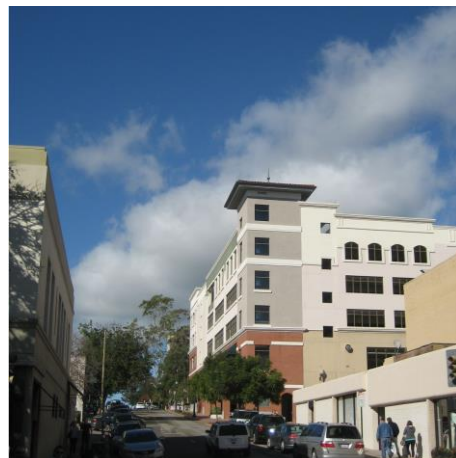
919 Palm St. Parking Structure
