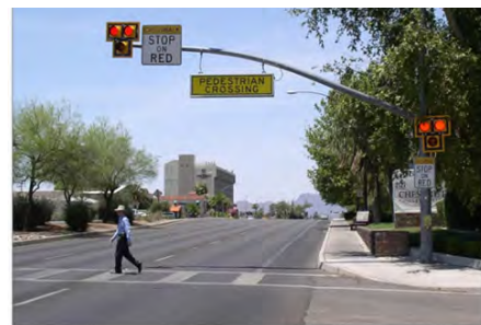
A pedestrian hybrid beacon (also known as the High intensity Activated crossWalk (or HAWK)) is a treatment that provides positive stop control in areas without the high pedestrian traffic volumes that typically warrant the installation of a signal
