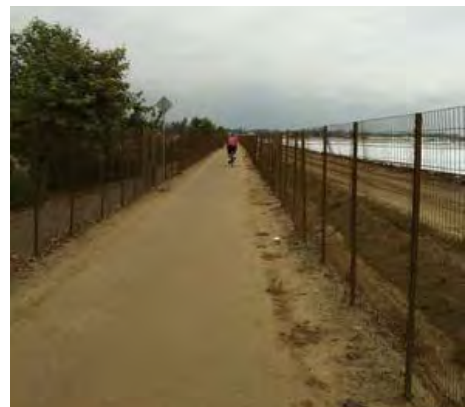
Wire mesh fencing along this Class I bike path along Arundell Barranca Channel in Ventura County deters path users from entering the adjacent agricultural lands and drainageway
