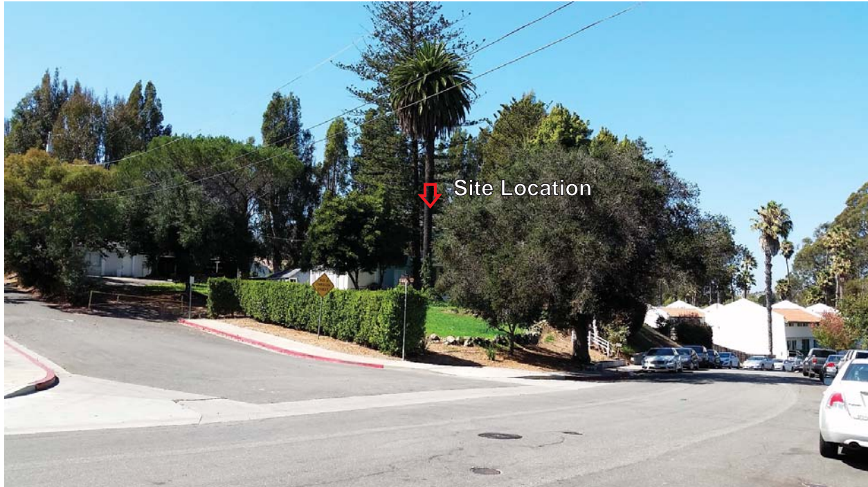
Key Viewpoint 5: Northwest-facing close-up view of project site from east side of Palomar Avenue at Luneta Drive.
