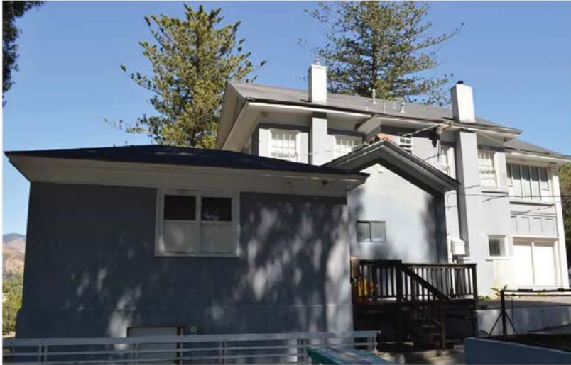
P5b.Description of Photo: View looking east at the rear (west) elevation of the residence. The two sequential additions are illustrated on the center and left side of the image.
