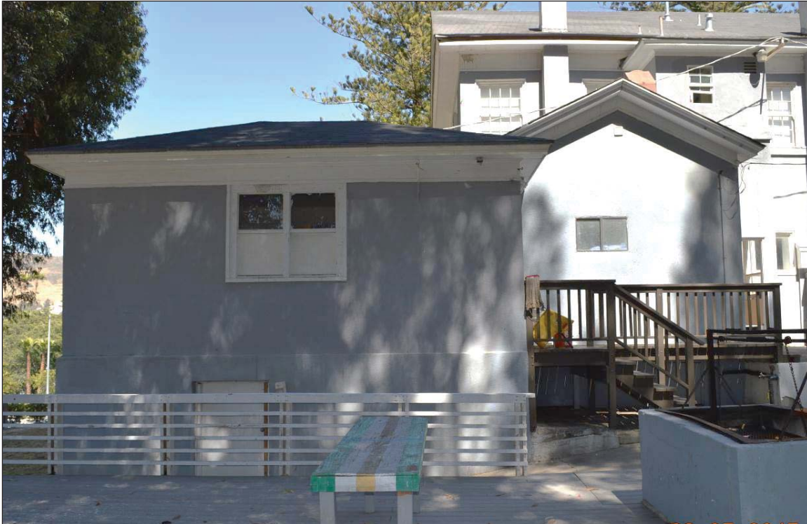
Figure 7-1 Two non-original additions to the rear of the Sandford House, looking west. The proposed project will demolish both additions.
