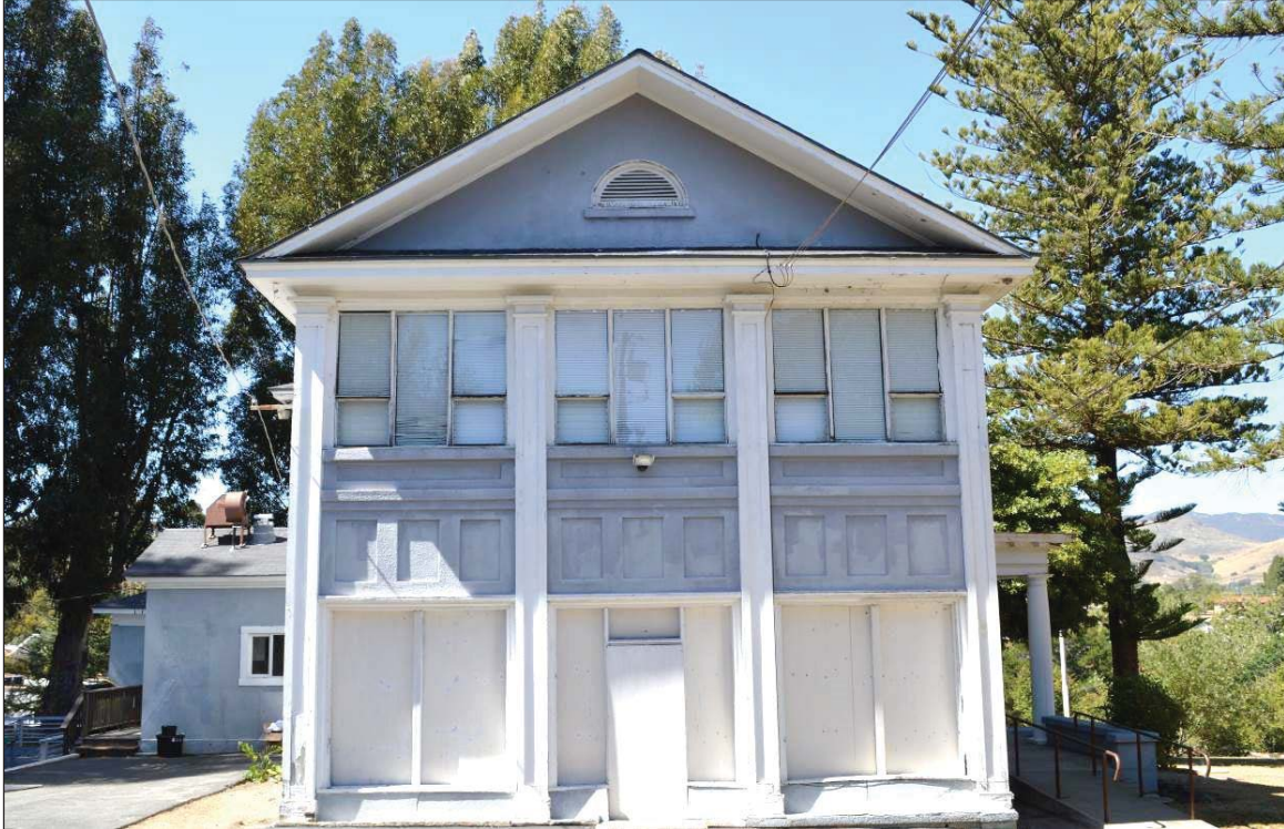
Figure 5-6 Two-story solarium on the south (side) façade of the Sandford House.
