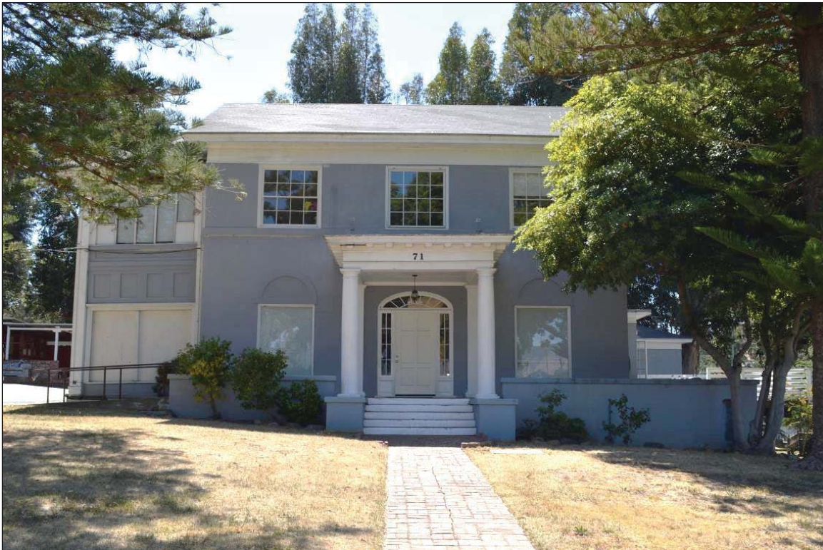
Figure 5-5 The Sanford House street-facing east façade.
