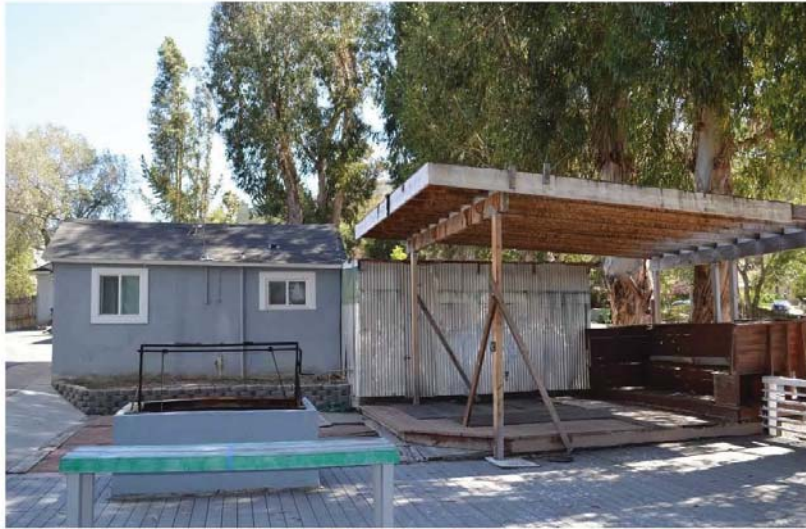
P5b.Description of Photo: View looking south at the north elevation of the second non-original accessory building and its rear addition. The covered patio and portion of the deck are also present in the image.
