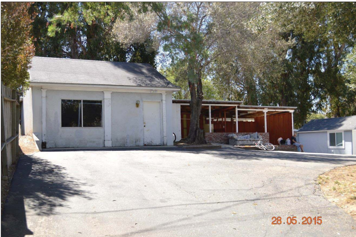
Figure 5-10 Enclosed garage with attached carport on the north façade.
