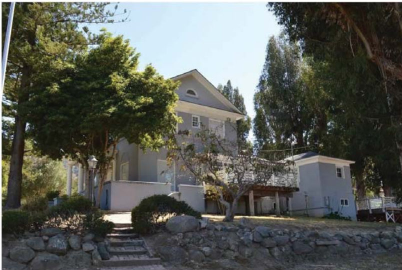
P5b.Description of Photo: View looking south at the side (north) elevation of the residence, with the second addition visible.
