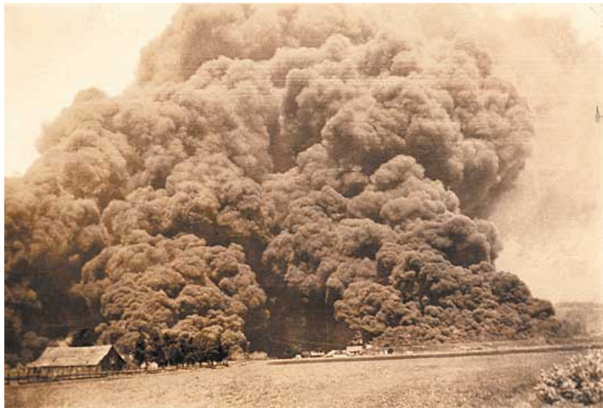
1926 Tank Farm Disaster
