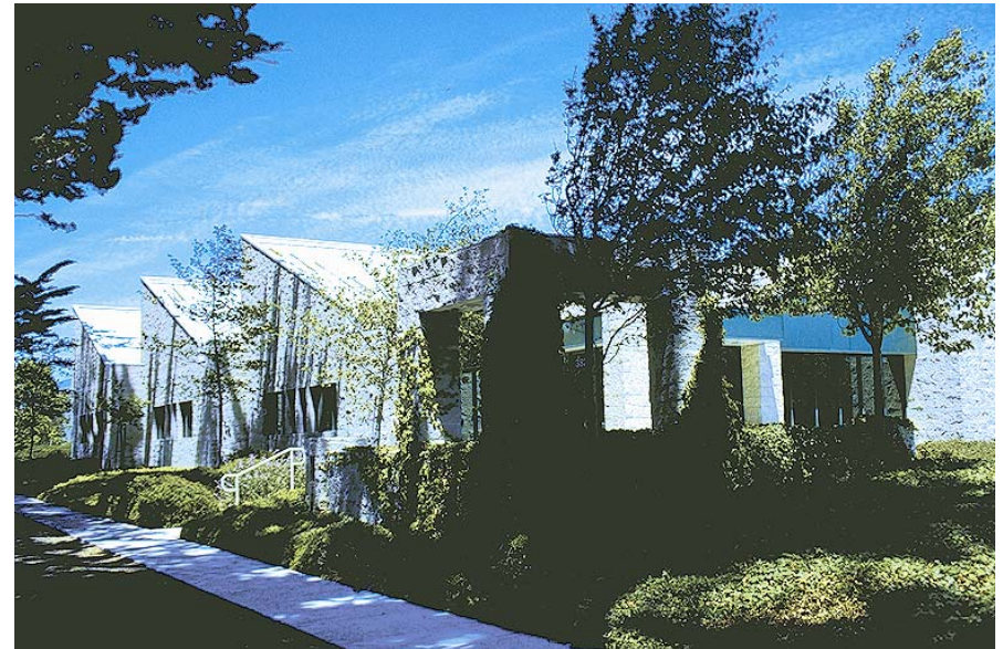
Roof forms should be varied to add interest and character to the area.
