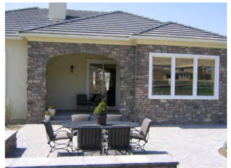
Offset windows prevent direct views from neighboring homes
