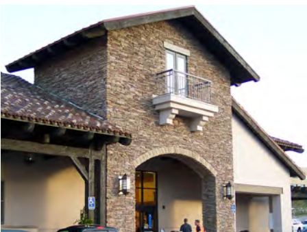
Change in building materials, pop-outs, and columns create shadow patterns and depth
