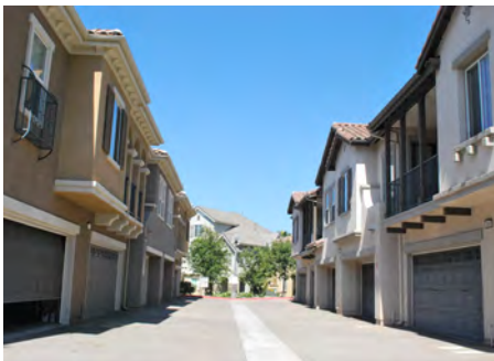
Garage doors were recessed and alley loaded to minimize visual impact
