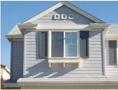
Accent trim such as sills and shutters make this house authentic to its architectural style
