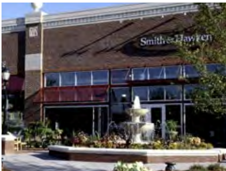
The use of brick complements the architectural style of this building
