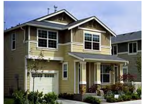
Architectural features such as porch, wood detailing, and siding enhance this home
