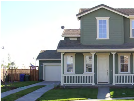
This home recessed the garage in order to help minimize visual impact of garage door
