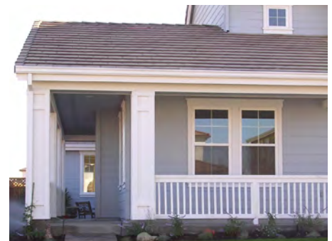
Offset windows and recessed second story to avoid direct sight lines and views
