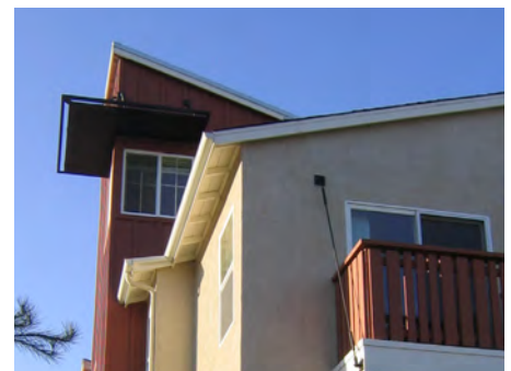
The use of a variety of roof pitches increases the visual quality of this home
