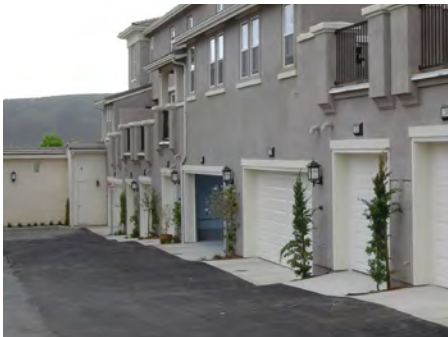
Garage entries were orientated away from street frontages to reduce visual impact
