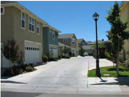
Detailed garage doors were used in these alley loaded garages
