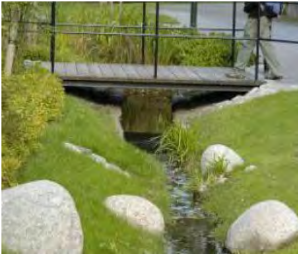
Low Impact Stormwater Control
