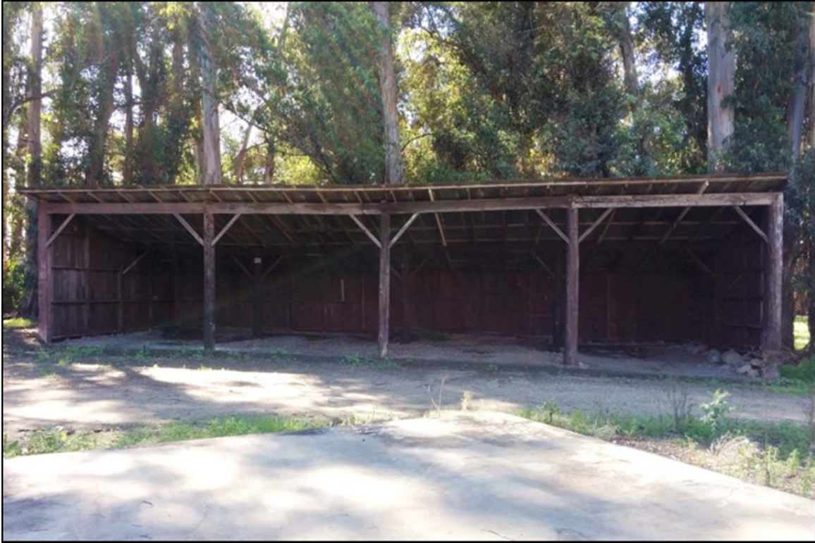
Photograph 11. Equipment storage building, north elevation, view to the south.
