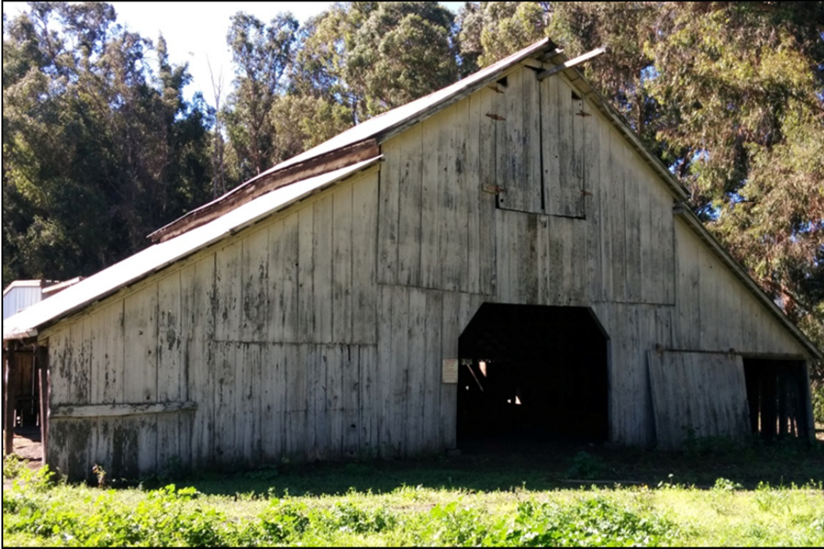
Photograph 10. Barn, north elevation, view to the southwest.
