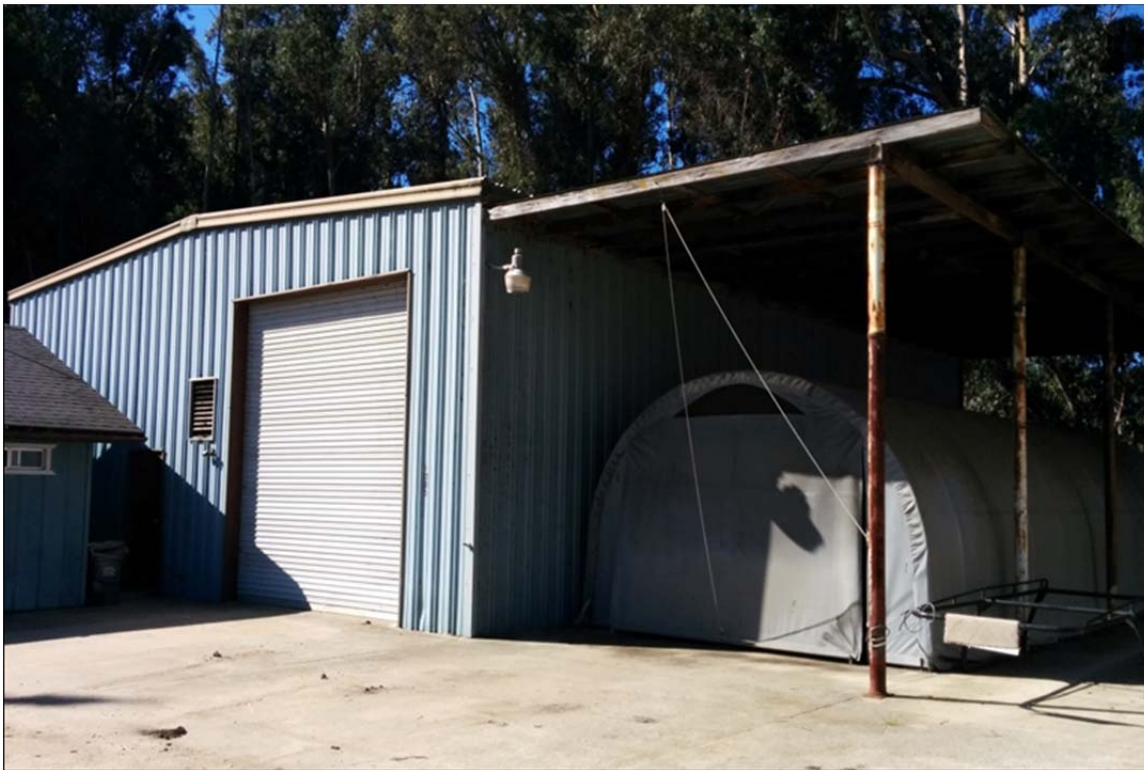
Photograph 12. Warehouse, east elevation, view to the southwest.
