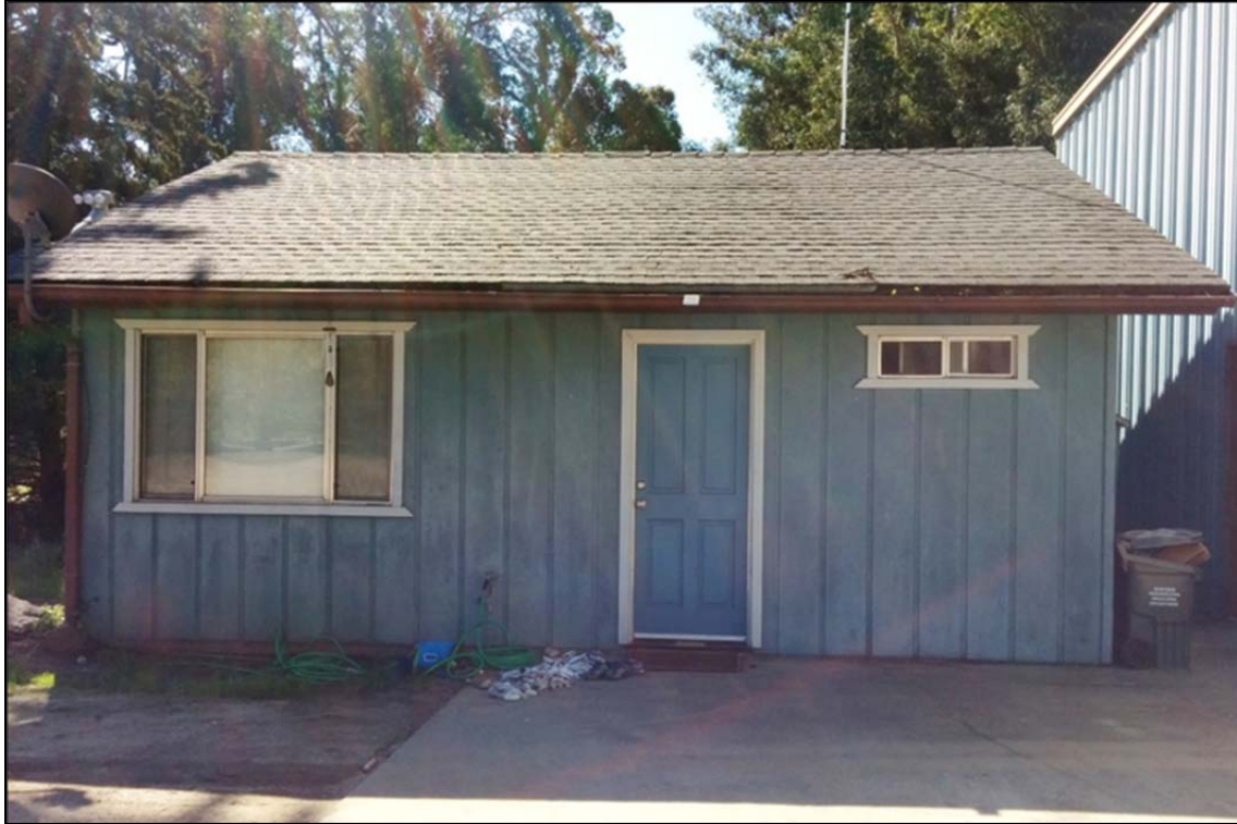
Photograph 7. Residence No. 3, view to the south.
