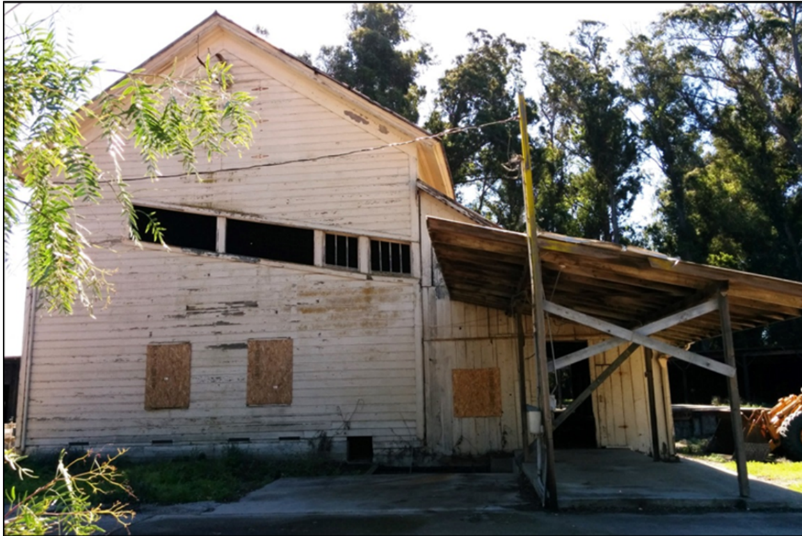
Photograph 13. Former spectator's barn/viewing stand, northwest elevation, view to the southeast.
