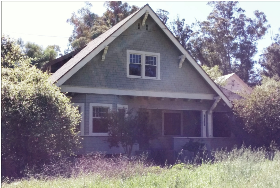
Photograph 5. Main residence, northwest elevation, view to the southeast.
