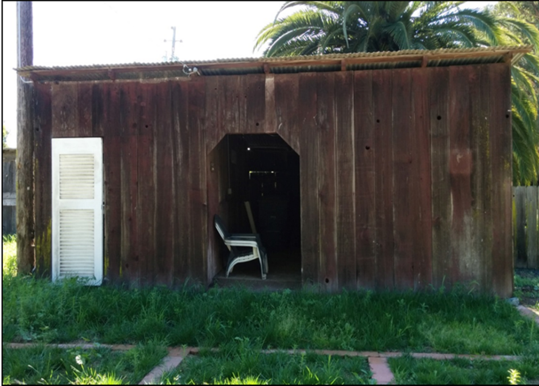
Photograph 9. Shed No. 2, northwest elevation, view to the southeast.
