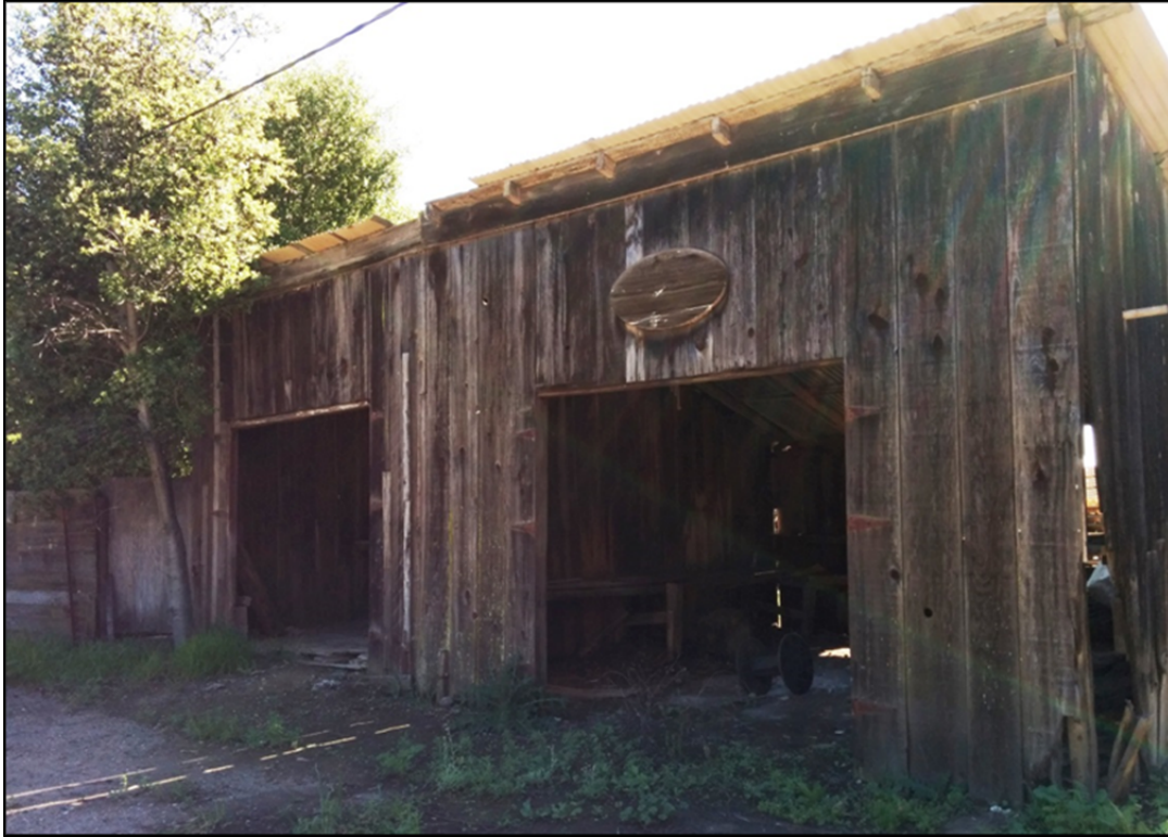
Photograph 8. Garage/shed, northwest elevation, view to the southeast.
