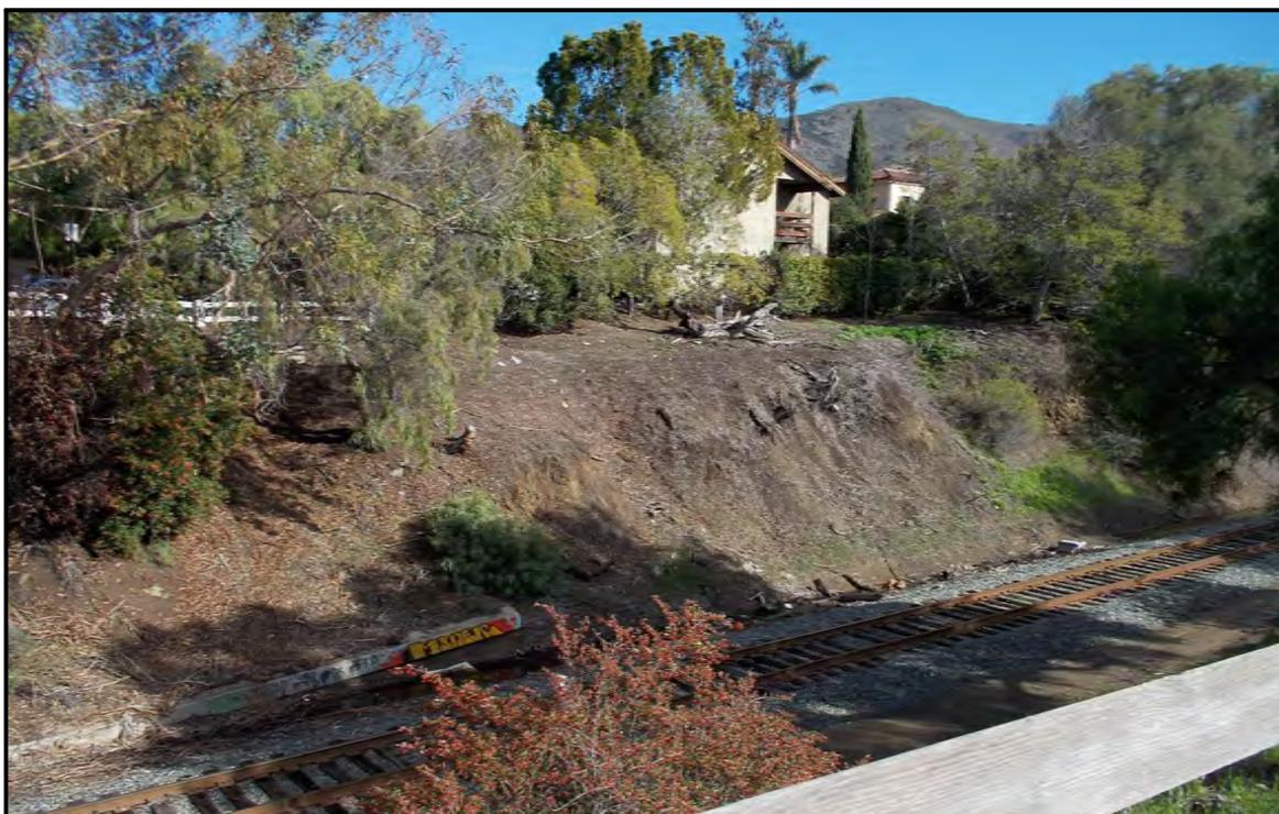
Photo 10: January 8, 2016. Facing aspect southeast from Pepper Lane is visible distressed vegetation along the eastern UPRR embankment.
