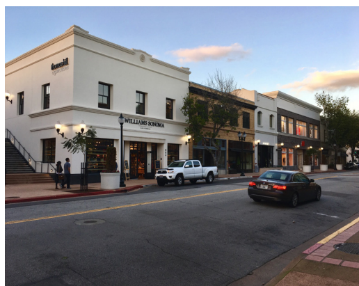
Chinatown Commercial Development Under Construction
