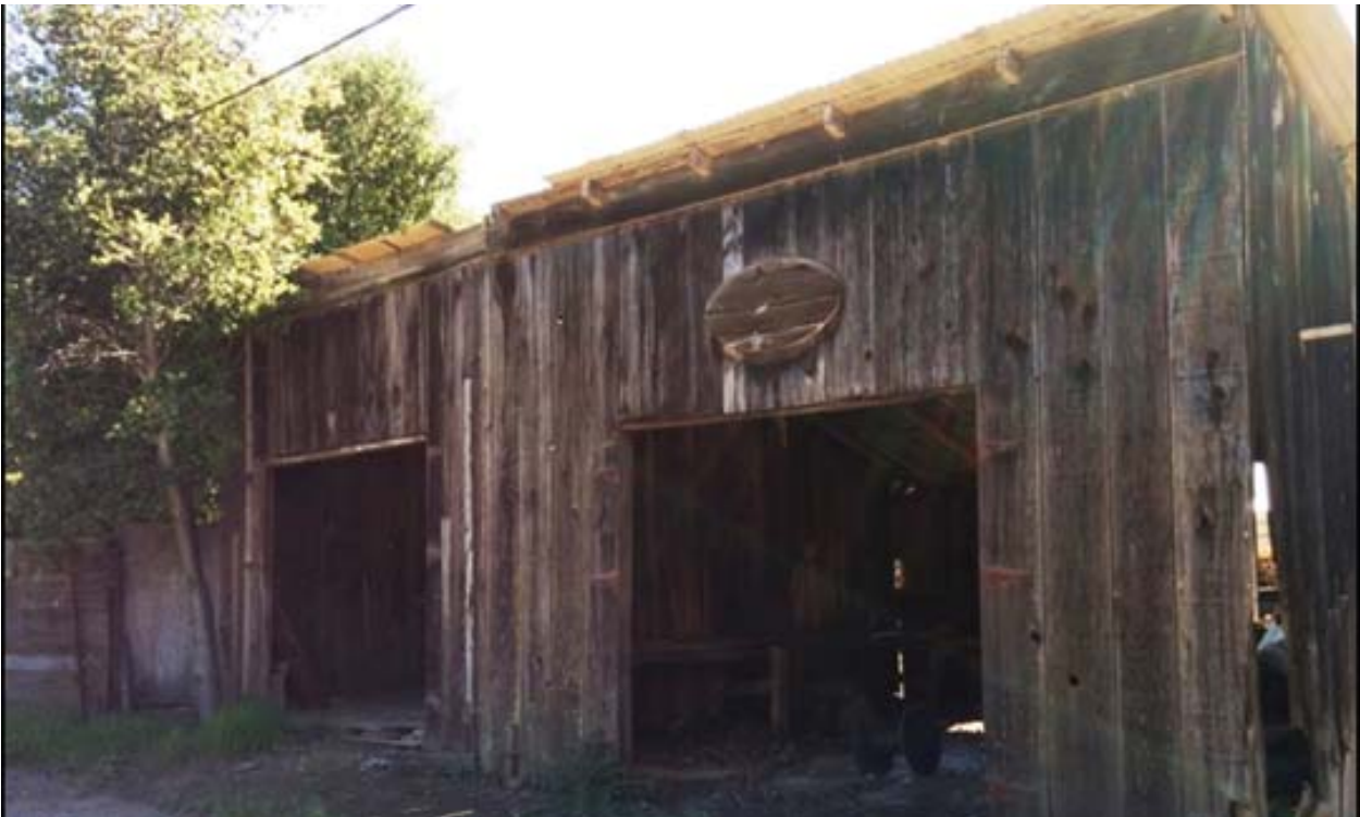
Photo 4: Garage/Shed, northwest elevation, view to the southeast.
