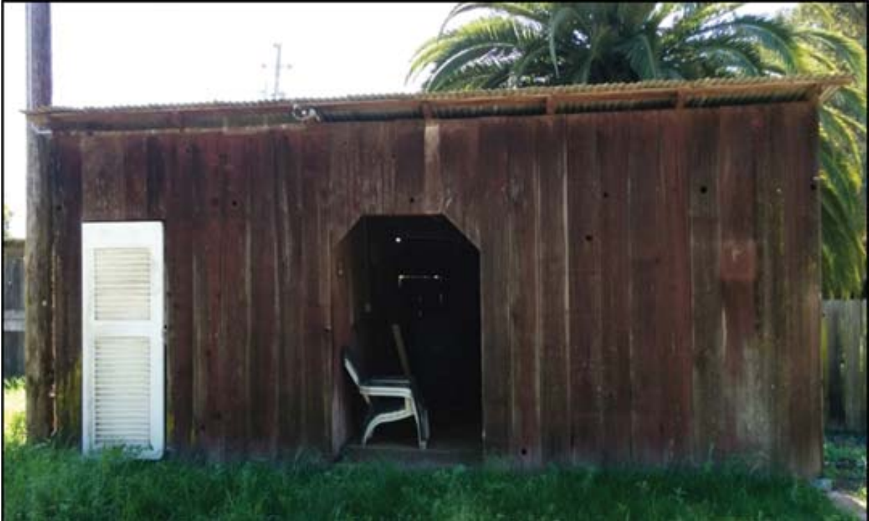
Photo 5: Shed #2, northwest elevation, view to the southeast.
