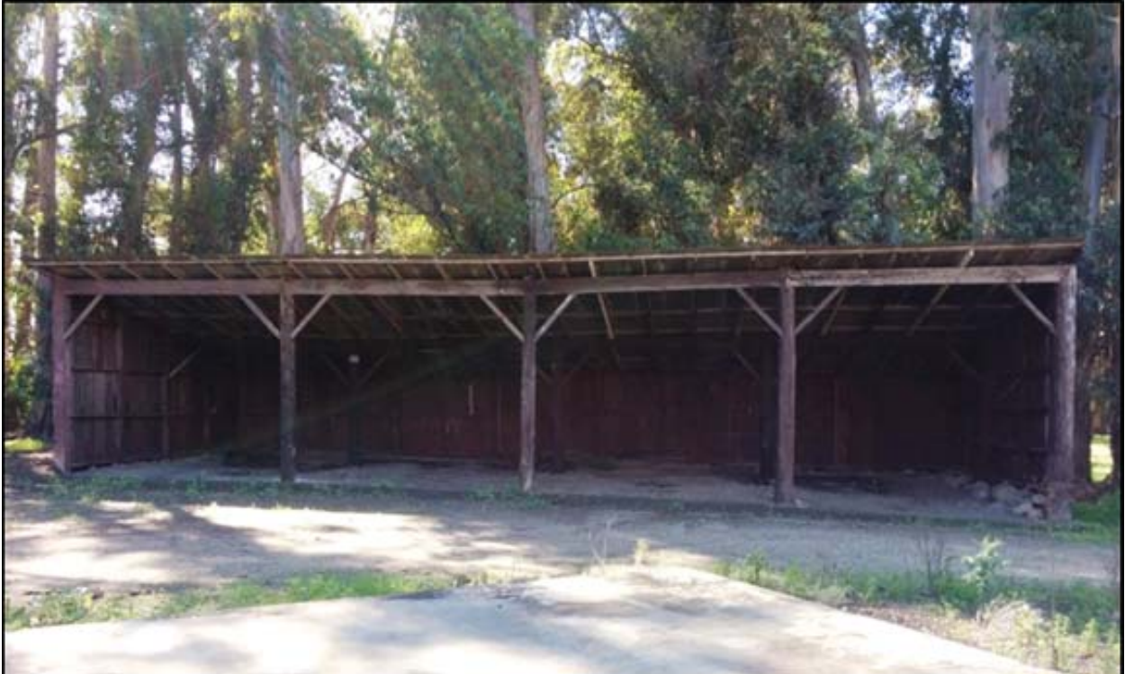
Photo 7: Equipment storage building, north elevation, view to the south.
