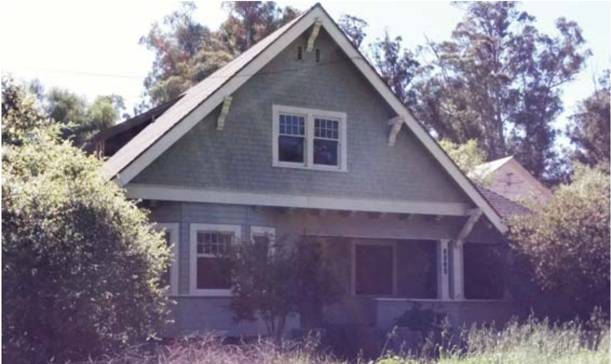
Photo 1: Main Residence (Residence #1), northwest elevation, view to the southeast.
