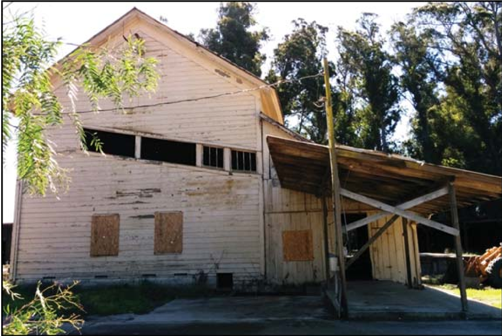
Photo 9: Former spectator's barn/viewing stand, northwest elevation, view to the southeast.
