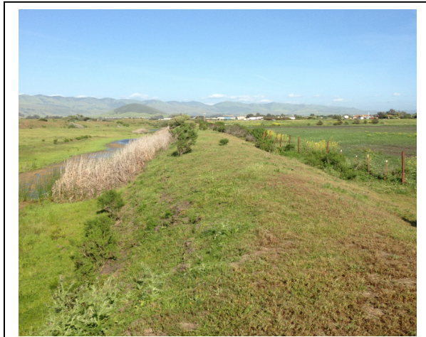
A 15- to 20-foot high berm separates the Chevron Tank Farm property from the northern boundary of the Project site.
