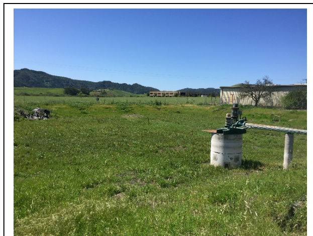
Within the western portion of Chevron Tank Farm property is a retention basin and associated pump.
