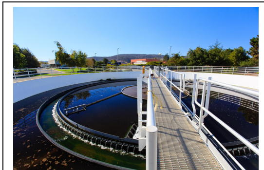
The WRRF removes solids, reduces the amount of nutrients, and eliminates bacteria in the treated wastewater before it is discharged to San Luis Obispo Creek.
