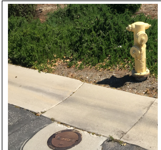
The access point to the water main on Earthwood Lane immediately north of the Project site. Currently, the water line is stubbed out within the Earthwood subdivision.
