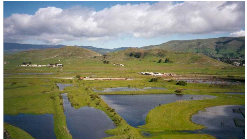
Swales and bermed enclosures on Chevron property now capture floodwaters.
