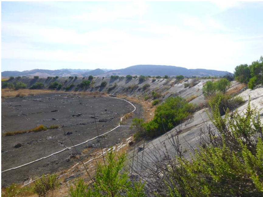
The 1926 fire burned so hot that parts of the concrete storage tank foundation turned to glass.
