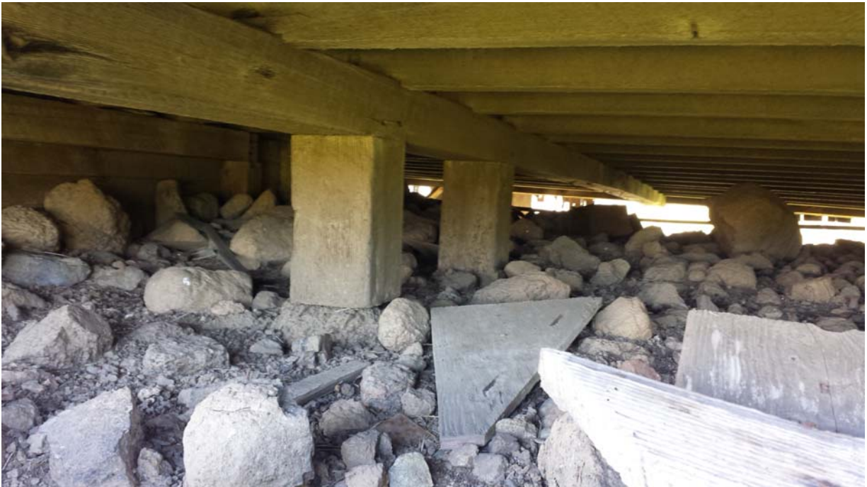
Figure 17 – Creamery House foundation
