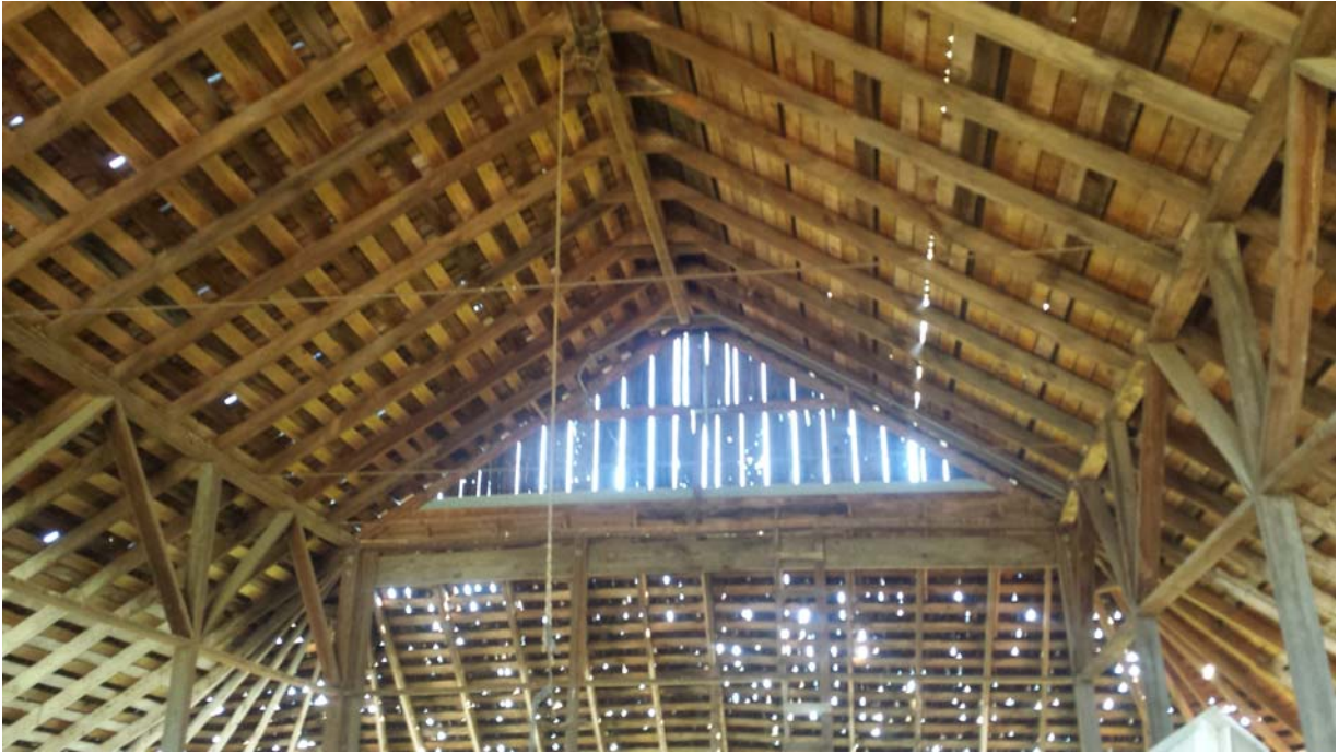
Figure 5 – Dairy Barn roof framing
