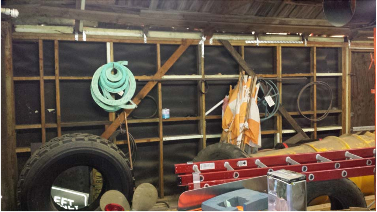
Figure 12 – Old Barn exterior wall framing
