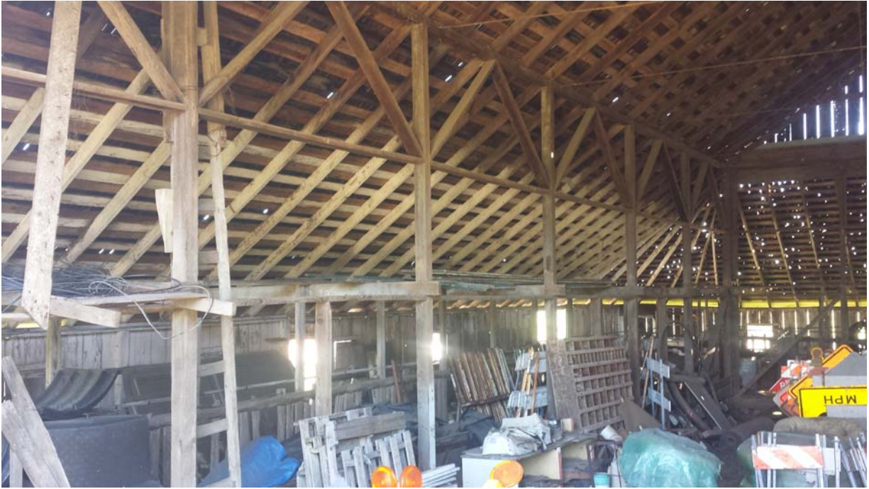
Figure 8 – Bracing at interior line of wood posts
