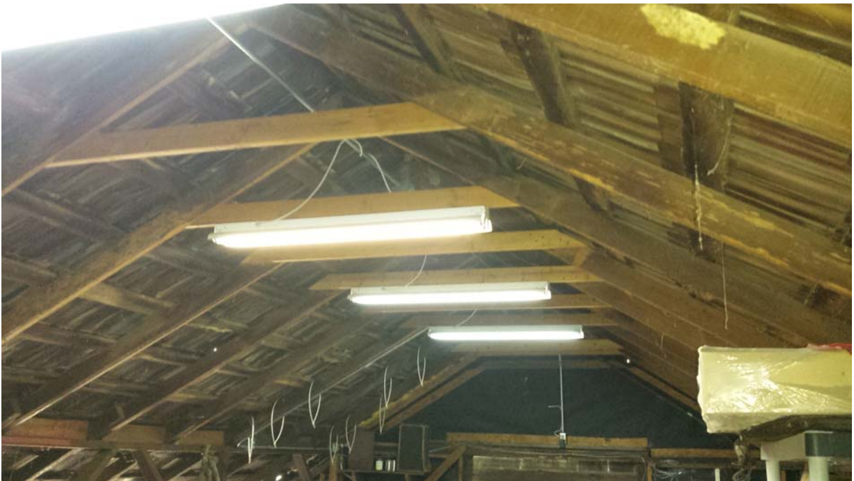
Figure 11 – Old Barn roof framing
