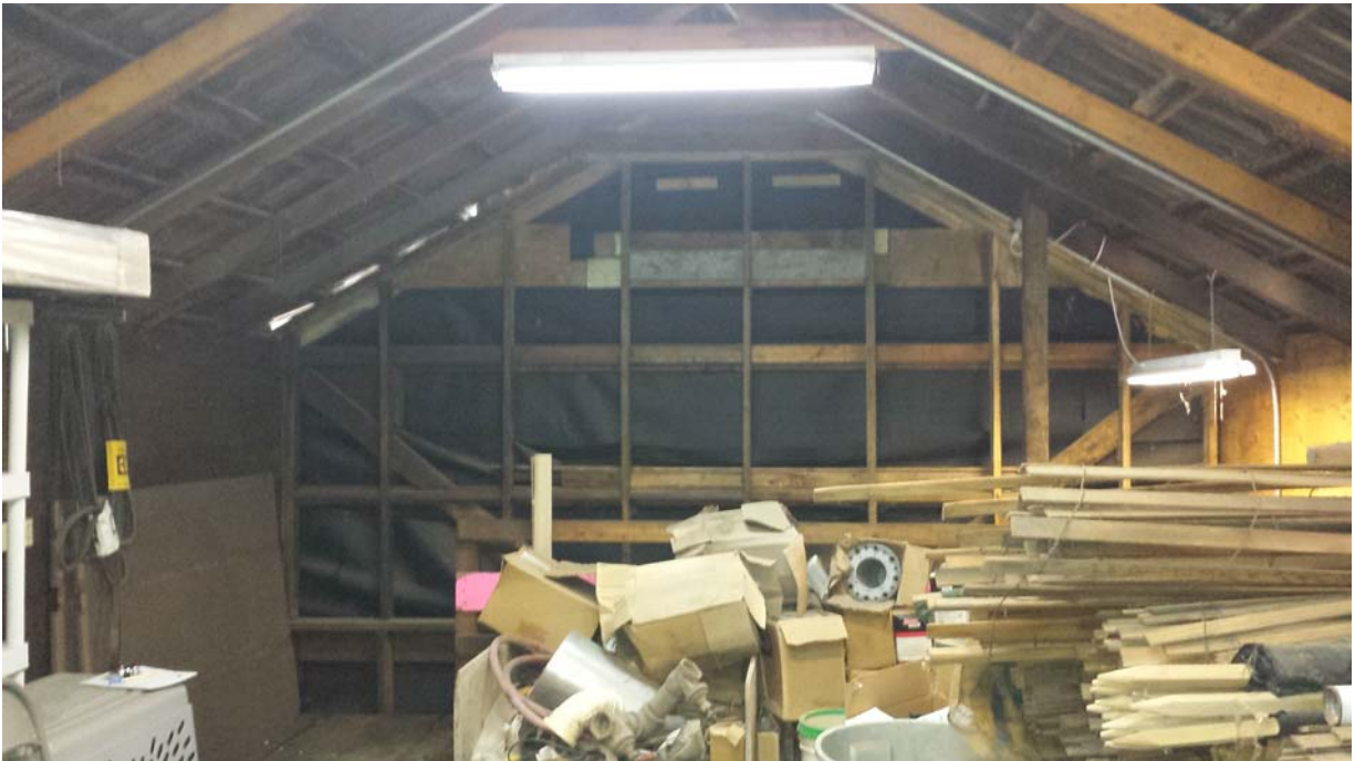
Figure 13 – Full-height plywood shear wall (left & right of photo)
