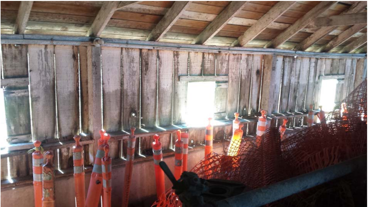
Figure 6 – Dairy Barn exterior wall framing
