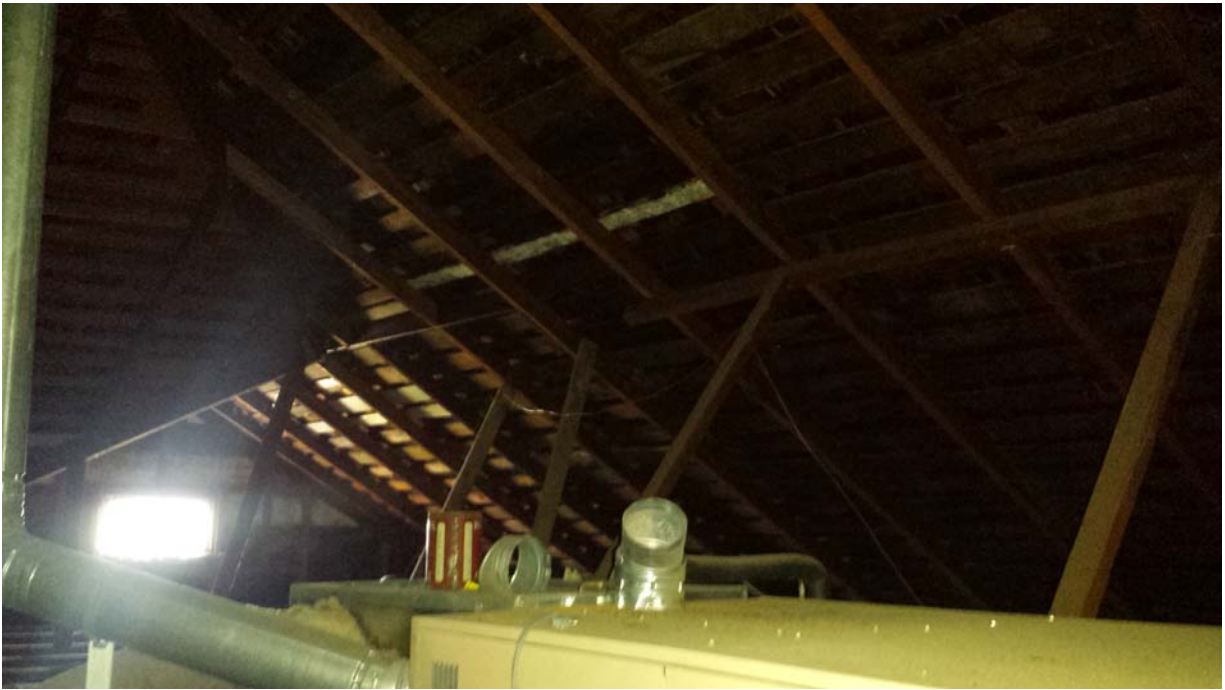
Figure 2 – Main House roof joists w/ mid-span bracing
