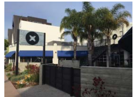
Renovated building on Monterey Street will help spur redevelopment
