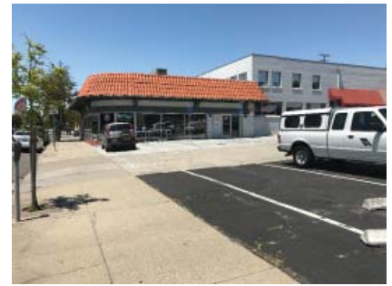
Location of new County office building; commercial or public use will help activate the street
