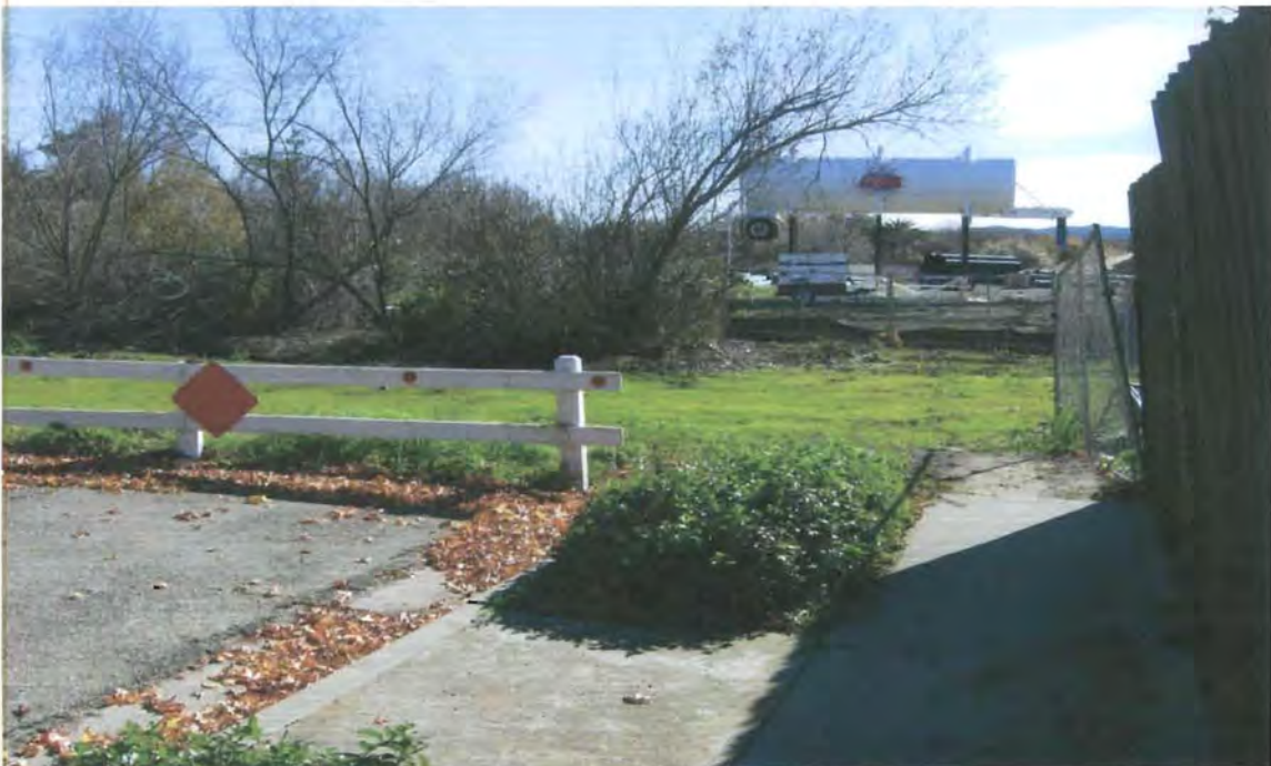
Figure 14. View of entry point onto the Bob Jones Trail from the end of Oceanaire Drive (Phase 1B). Construction still underway in background.
