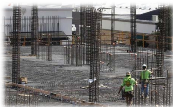
Chinatown Hotel SLO Under Construction
