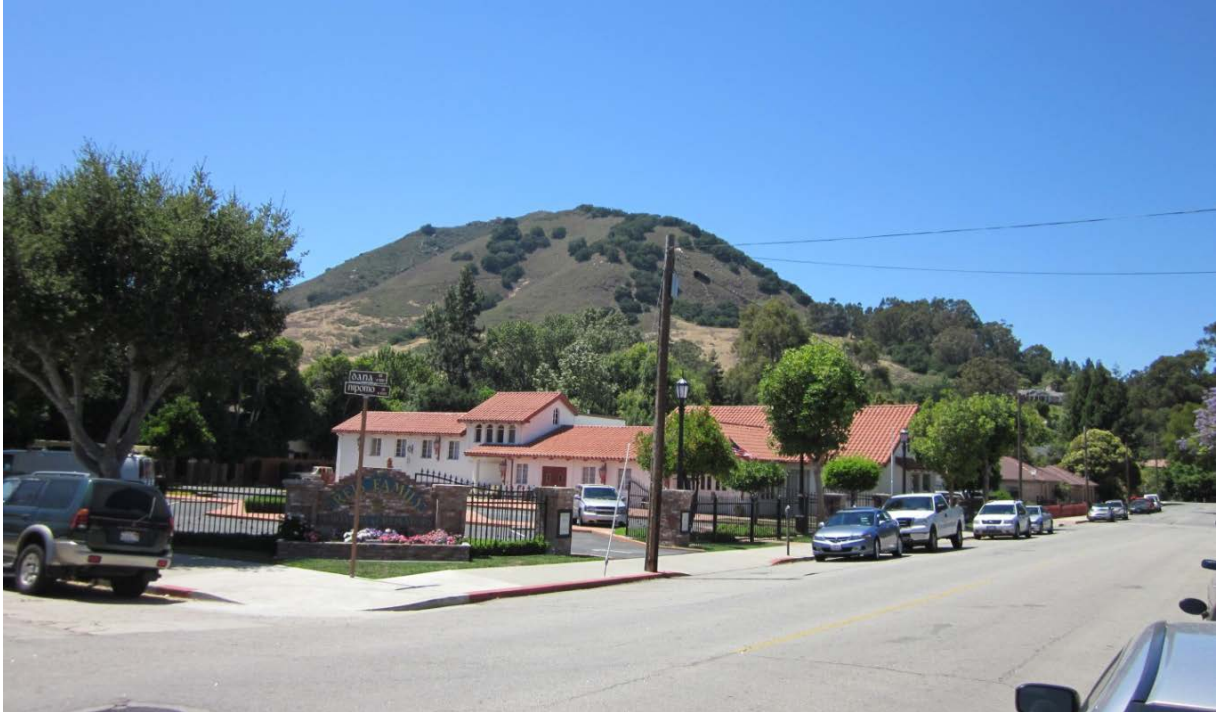
Photograph 3. View of historic Harmony Creamery (Reis Family Mortuary) from project site at the corner of Monterey and Nipomo streets looking northwest
