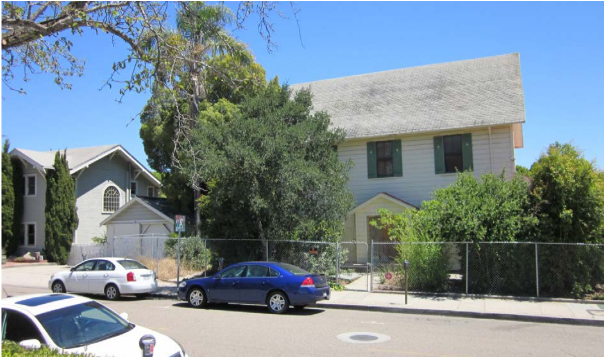
Photograph 1. View of 667 Monterey Street from project site looking south
