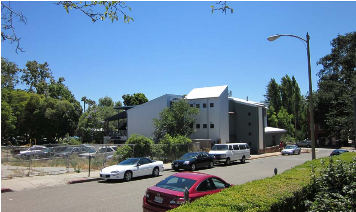
Photograph 4. View of San Luis Obispo Children's Museum from project site looking southwest
