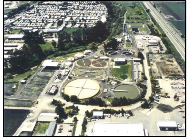
City wastewater treatment facility on Prado Road
