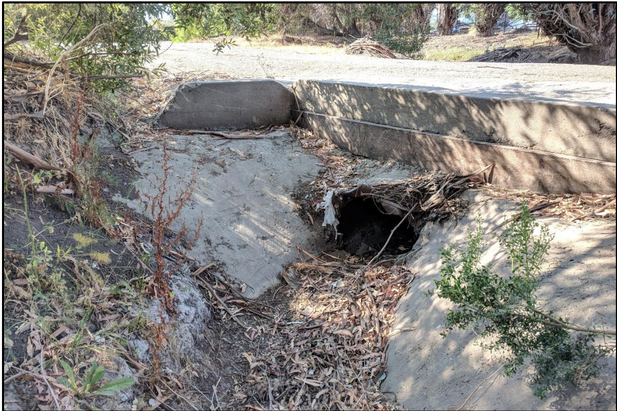
Figure 9 Eastern Creek Corridor, Facing South
