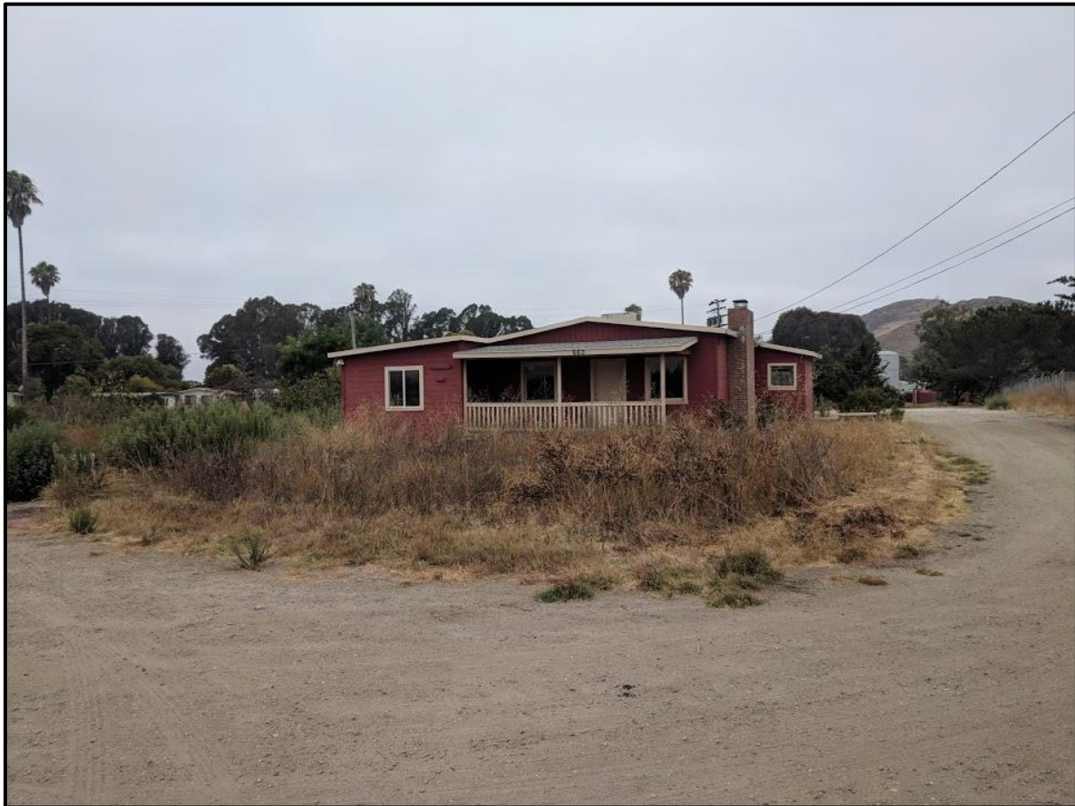
Figure 10 660 Tank Farm Road
