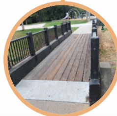
MEADOW PARK PATHWAY MAINTENANCE AND PEDESTRIAN BRIDGE REPLACEMENT SPRING 2019
