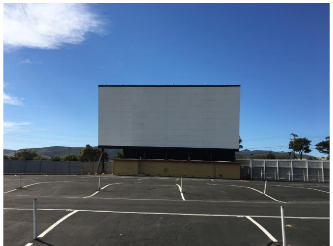
Movie screen and building supporting it, view to the west.
