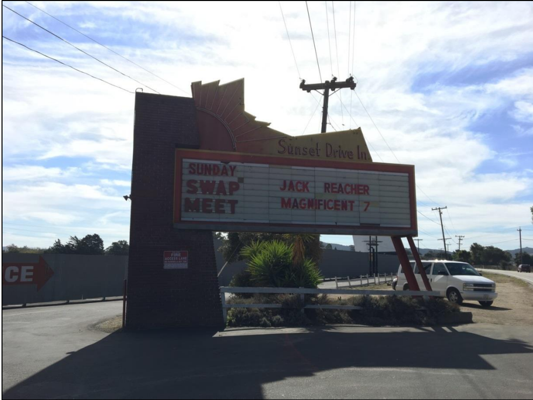
Figure 10. Marquee, facing south.
