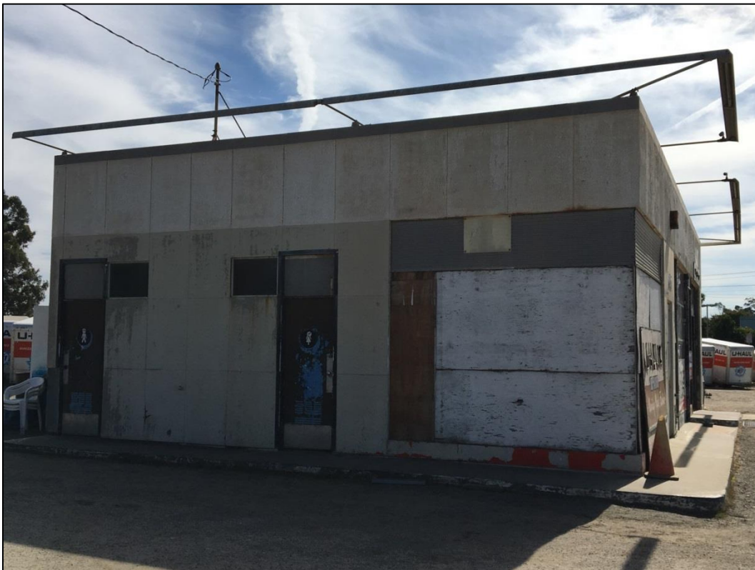
Figure 6. Northwest elevation of building.
