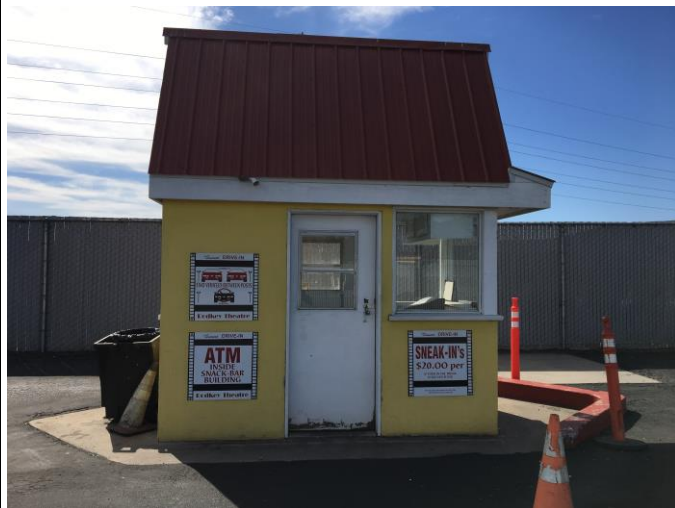
Ticket booth, view to the south.
