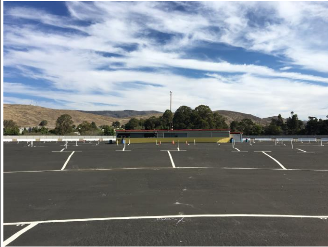
Detail of auto parking area, view to the southwest.
