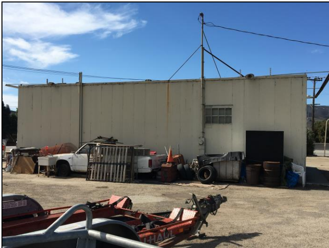
East elevat., looking west.
