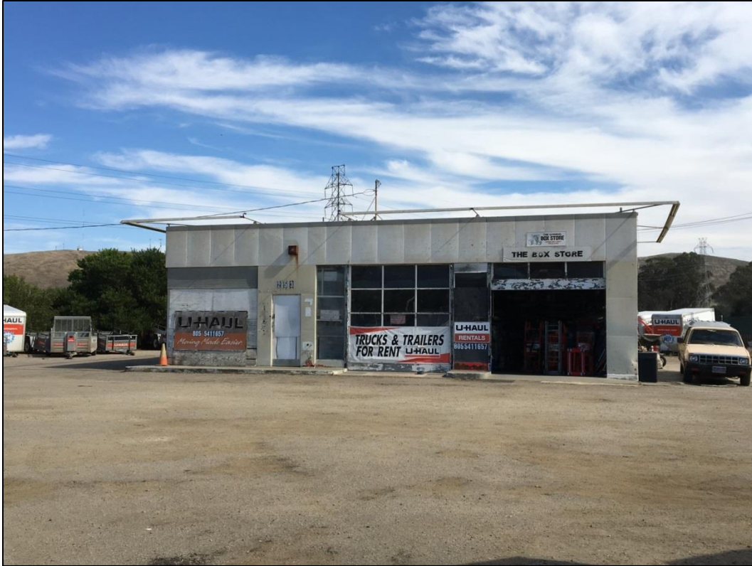
Figure 5. Southwest elevation of building.
