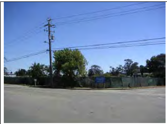
21. SLO City Water Treatment plant, south of property.
