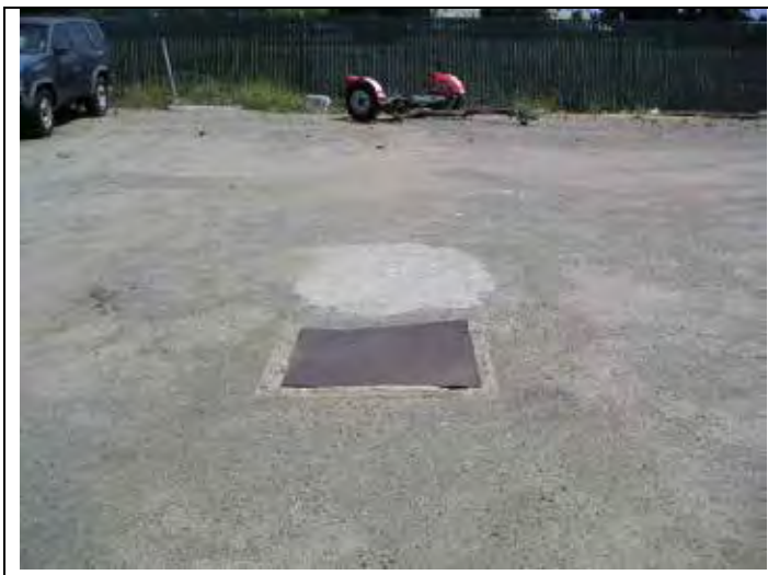
7. View of septic tank at northeast corner of U-Haul parcel.
