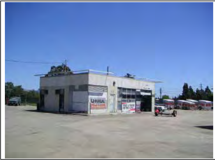
1. Front of U-Haul building, as viewed facing northeast.
