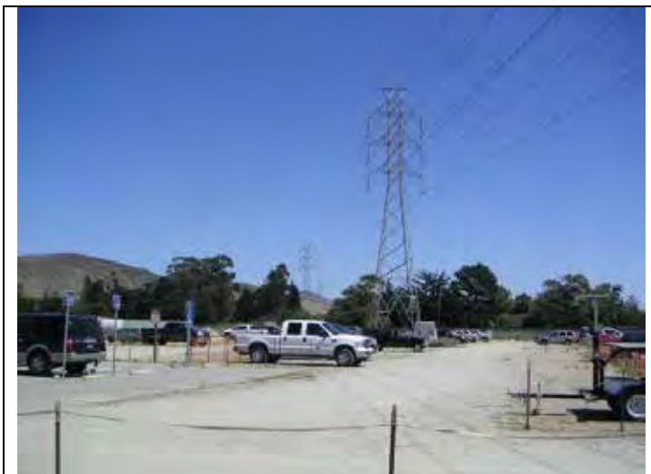
10. View of Topaz Solar Farm parking lot.
