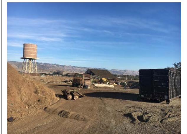
The Specific Plan area is largely undeveloped and used for grazing. However, the northwestern portion of the site is developed with historic dairy ranch buildings and a permitted quarry used for storage of construction materials.
