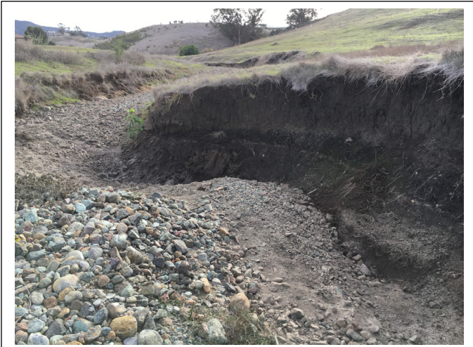
Froom Creek traverses the Project site within a narrow channel composed of rock, gravel, and sand. Evidence of eroded, undercut banks from high-velocity flows was observed onsite (January 2018)
