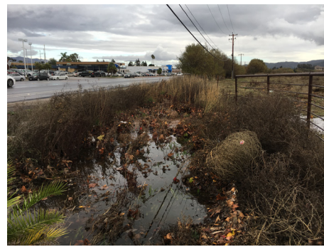
The man-made drainage ditch adjacent to LOVR conveys stormwater runoff from adjacent development to the north and east. Prolonged ponding of runoff has resulted in the establishment of high-quality wetland and riparian habitats.
