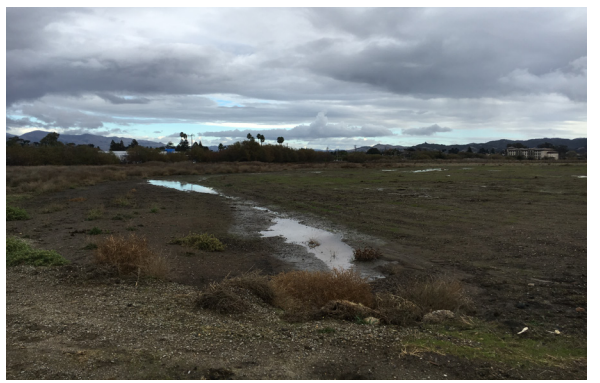
Runoff from adjacent Irish Hills Plaza flows to onsite detention features on the Project site, including a 3.2-acre basin, and creates pooling in a former infiltration area adjacent to the existing driveway (pictured).
