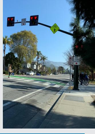
PHB's provide an effective solution for improving safety for pedestrians and bicyclists, with less delay to drivers.
