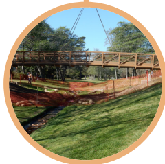
MEADOW PARK PEDESTRIAN BRIDGE REPLACEMENT COMPLETED APRIL 2020
