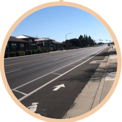
SOUTH BROAD STREET ROAD REHABILITATION COMPLETED AUGUST 2019
