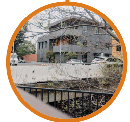
MARSH STREET BRIDGE REPLACEMENT DECEMBER 2020
