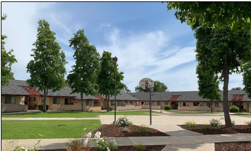
Figure 2: Poinsettia Street Apartments
