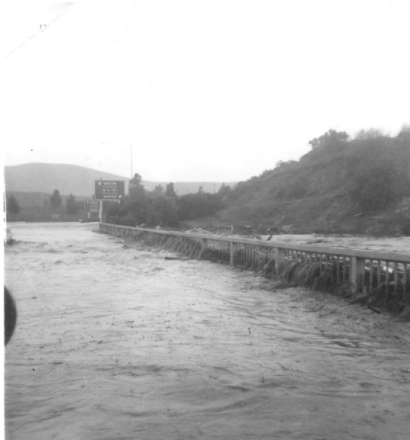
Marsh Street Bridge
