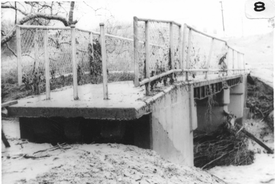
Andrews St. Footbridge
