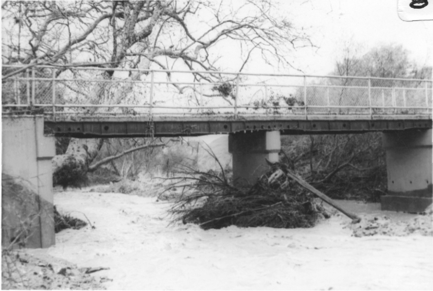
Andrews St. Footbridge
