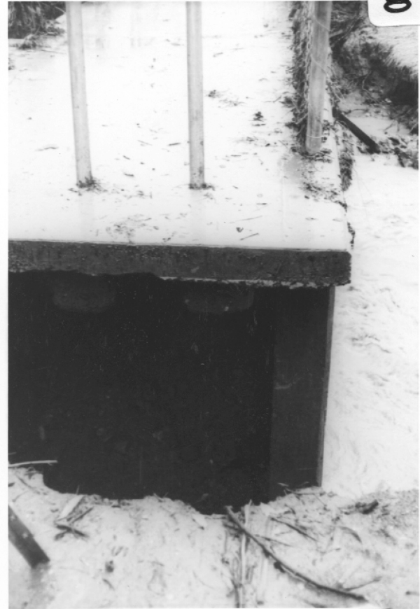
Andrews St. Footbridge
