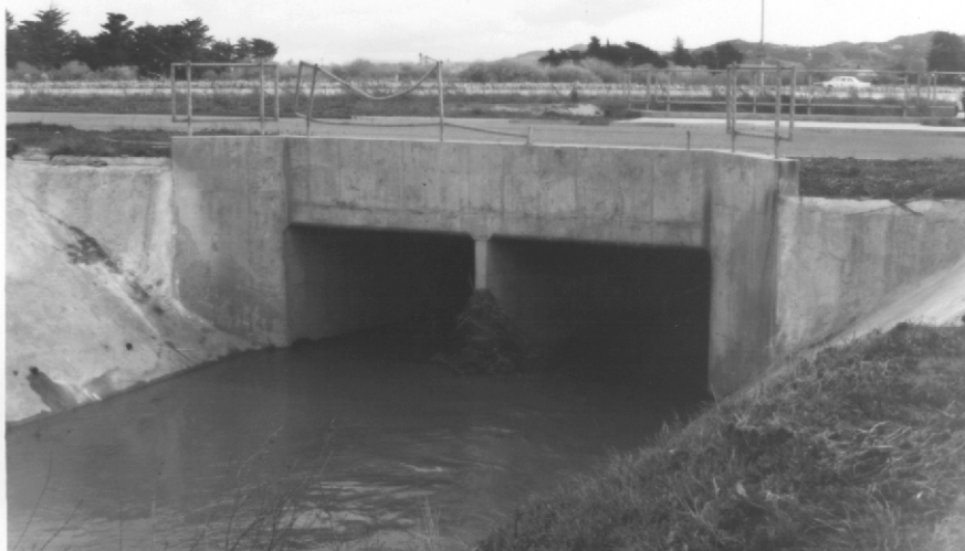
Tract 347 (Calle Joaquin culvert)
