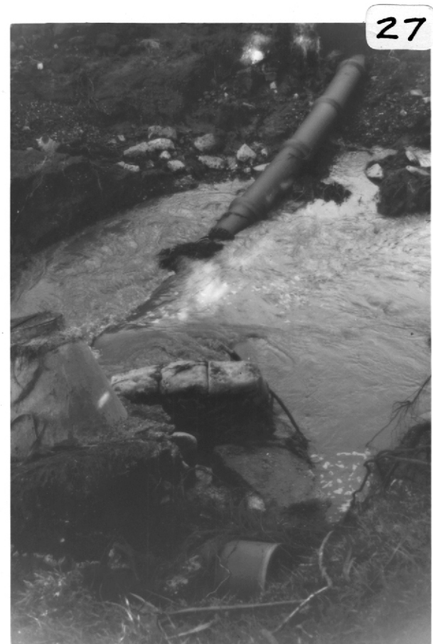
Laguna Lake Outlet (broken sewer)
