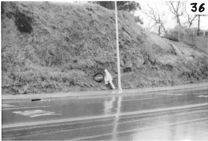
Johnson Avenue Underpass (sewerline)
