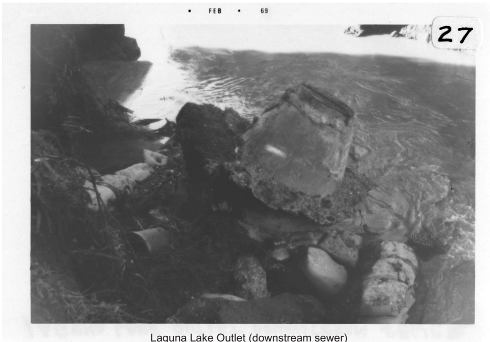
Laguna Lake Outlet (downstream sewer)
