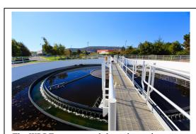
The WRRF removes solids, reduces the amount of nutrients, and eliminates bacteria in the treated wastewater before it is discharged to San Luis Obispo Creek.
