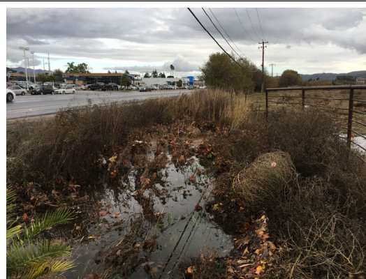
The man-made drainage ditch adjacent to LOVR conveys stormwater runoff from adjacent development to the north and east. Prolonged ponding of runoff has resulted in the establishment of high-quality wetland and riparian habitats.
