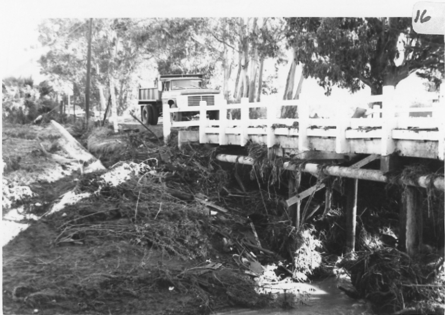
Elks Lane Bridge
