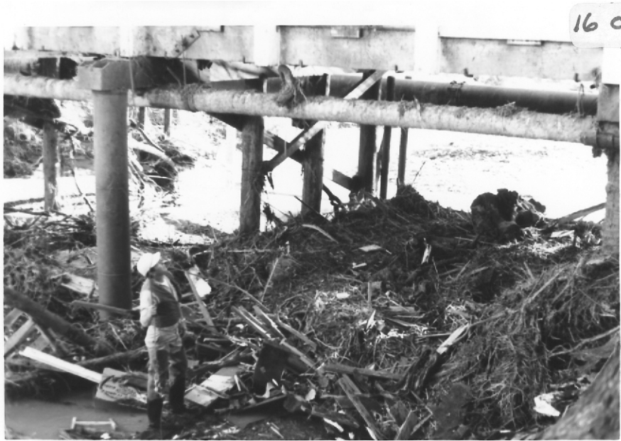
Elks Lane Bridge at San Luis Creek
