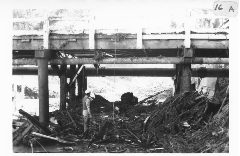
Elks Lane Bridge at San Luis Creek
