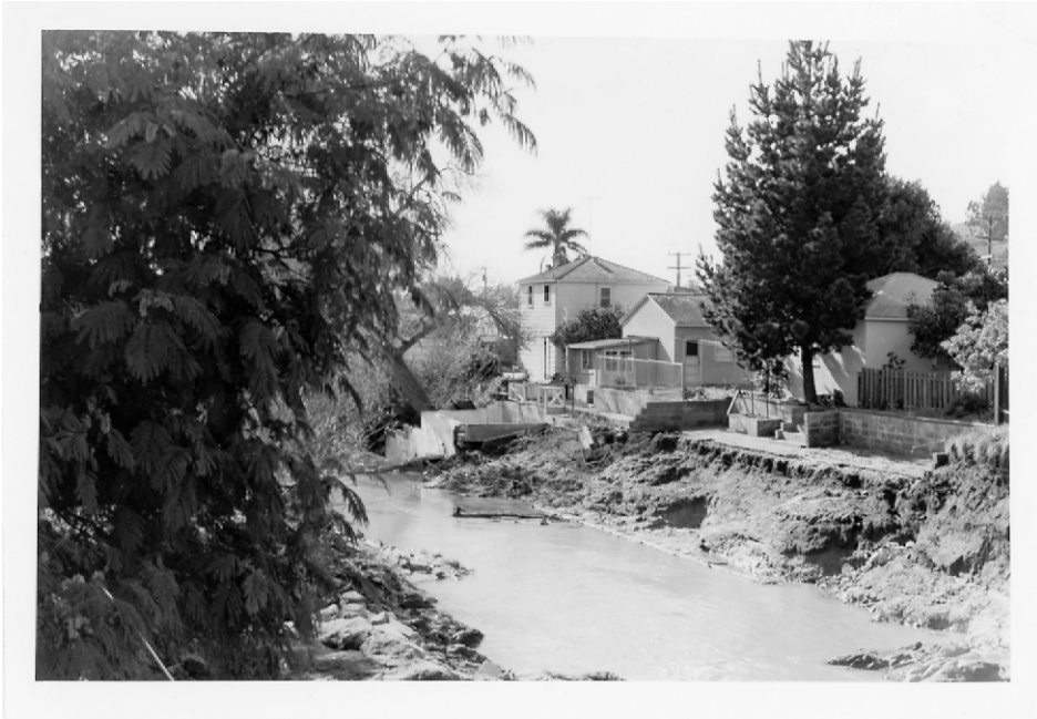
Erosion of land and damaged patios along Stenner creek
