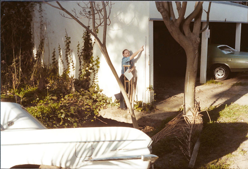
24. (cont'd) High water marks
