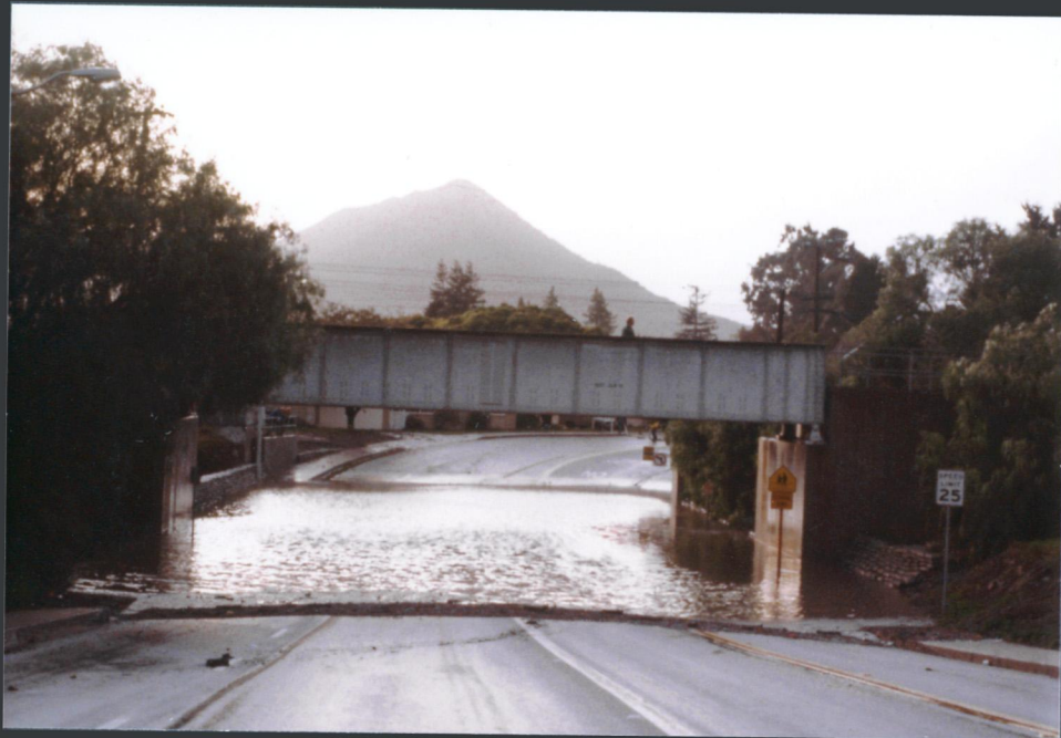
27. Johnson Avenue underpass
