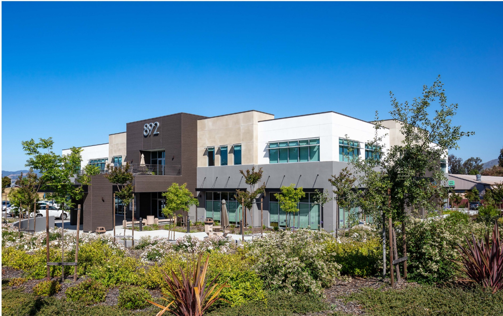
Figure 4. Image of Similar Adjacent Structure.
