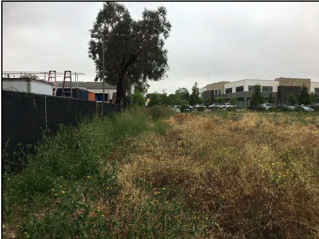
Photo 8. Densely vegetated swale that conveys flow from 12-inch culvert at the northeast corner of the Survey Area (Aspect: East).
