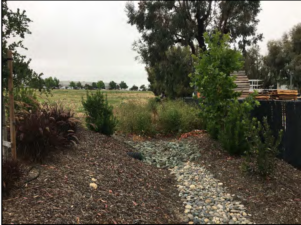
Photo 7. 12-inch culvert on the adjacent parcel at the northeast corner of the Survey Area (Aspect: West).
