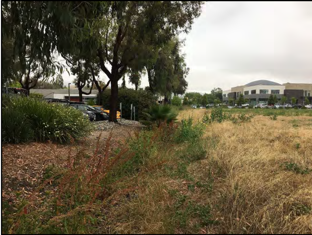
Photo 5. Unnamed tributary at the northern property boundary prior to entering the 48-inch box culvert (Aspect: East).
