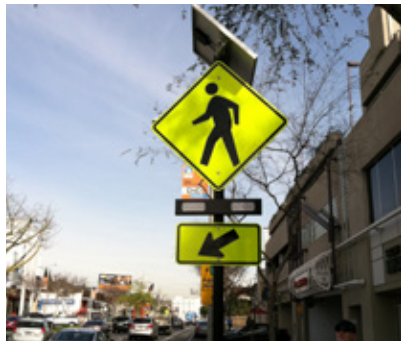
Rectangular Rapid Flashing Beacon
