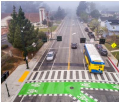
Green Bike Lane Markings
