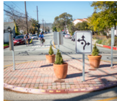
NEIGHBORHOOD TRAFFIC CIRCLE
