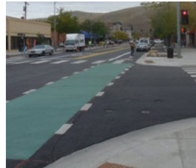
GREEN BIKE LANE MARKINGS
