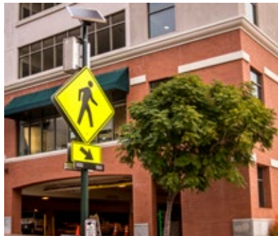
Rectangular Rapid Flashing Beacon
