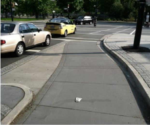
Clear sight lines at intersections and driveways for people on bikes and people driving are an important aspect of this design.
