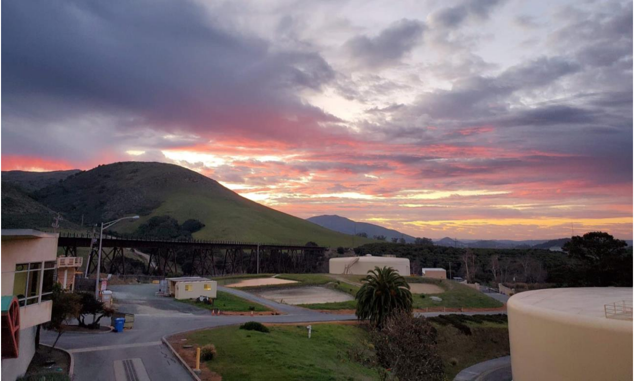
Stenner Canyon Water Treatment Plant.
