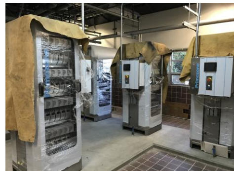
Installation of new Ozone Generators.
