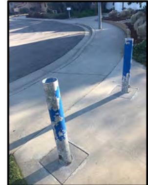
*Figure 14a. Paint chipping on bollards*
