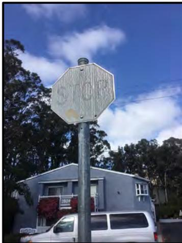
*Figure 13a. Faded Stop sign*
