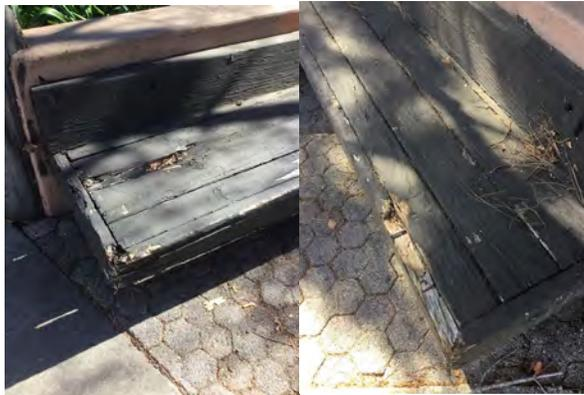
2. A (2) bench had either some larger cracks or chips but did not affect the feel or safety of the bench for concrete, or for expanded metal it had some damage or some paint chipping but did not affect the safety of the table.
