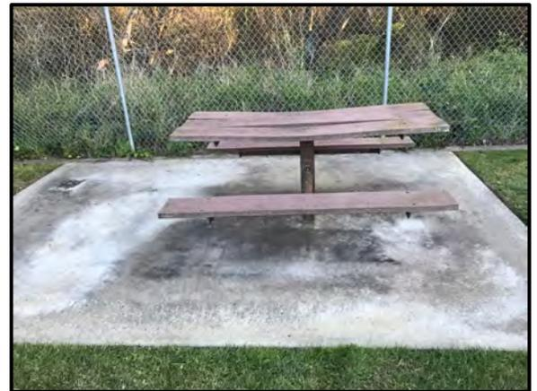
*Figure 28b. Warped picnic table*
