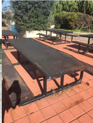
2. A (2) picnic table had either some larger cracks or chips but did not affect the feel or safety of the table for concrete, or for expanded metal it had some damage or some paint chipping but did not affect the safety of the table.
