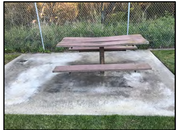
Figure 28b. Warped picnic table
