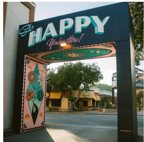
Archway to Happiness - Marsh Parking Garage
