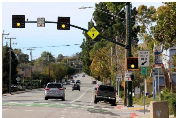
New RRFB Beacon installed at Monterey & Buena Vista
