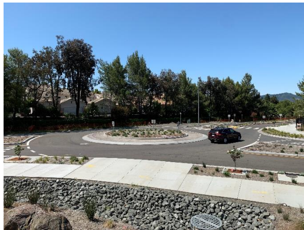
New Roundabout at Righetti Ranch Rd & Tank Farm Rd
