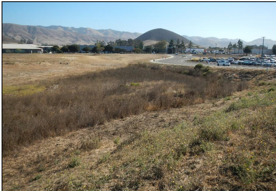
Photo 4. Looking east at the upstream portion of the drainage where it enters the survey area through a culvert under Aero Drive (11-11-19).
