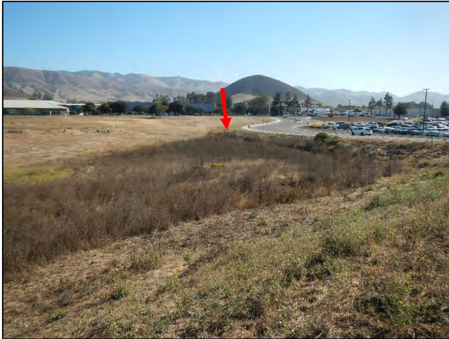
Photo 1. View east of drainage where it enters the survey area through a culvert (red arrow) under Aero Drive (10-03-19).
