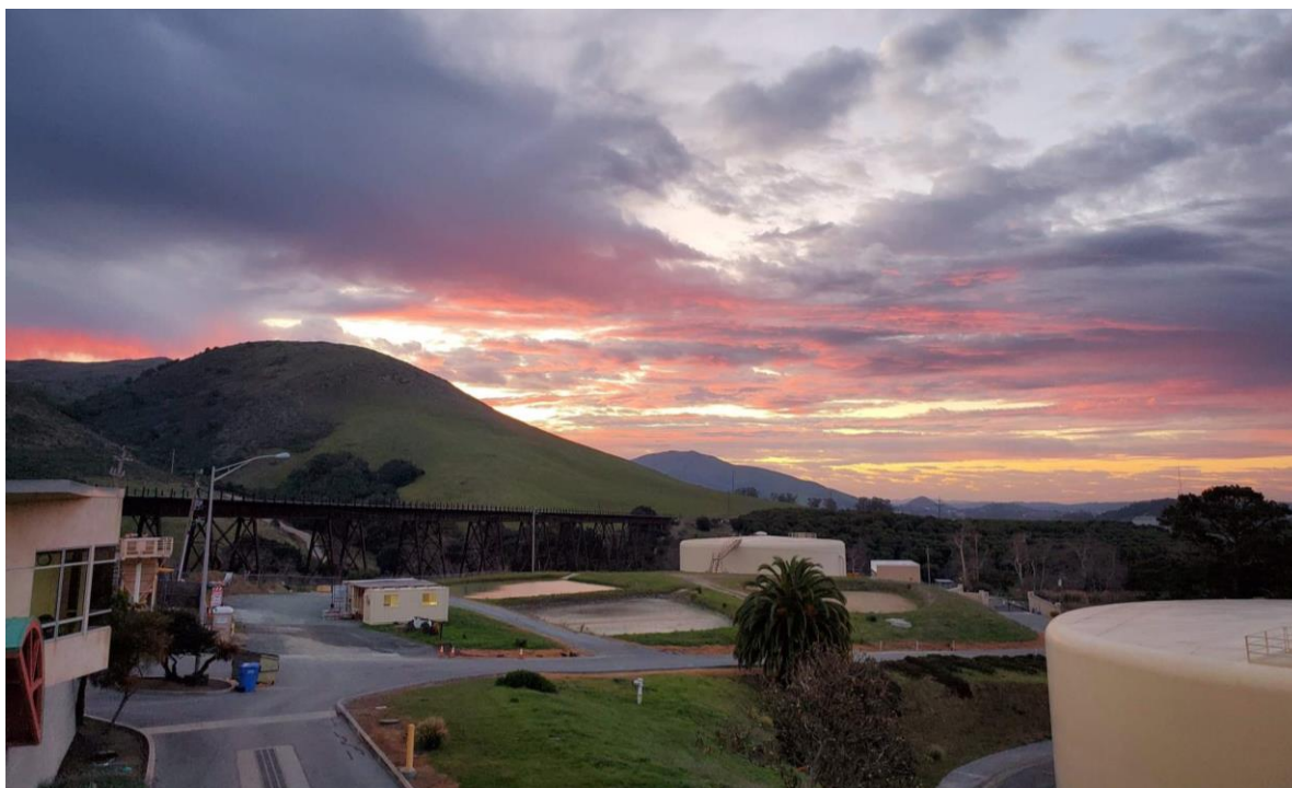
City of San Luis Obispo Water Treatment Plant, 2020
