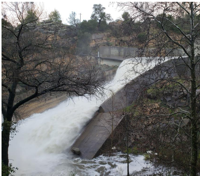
Salinas Dam spillway, February 2019.
