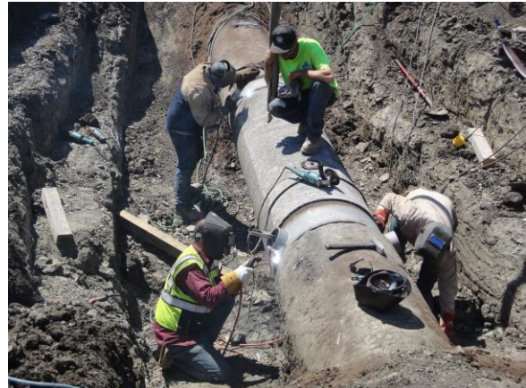
30-inch Whale Rock Pipeline Repair Conducted in June 2017
