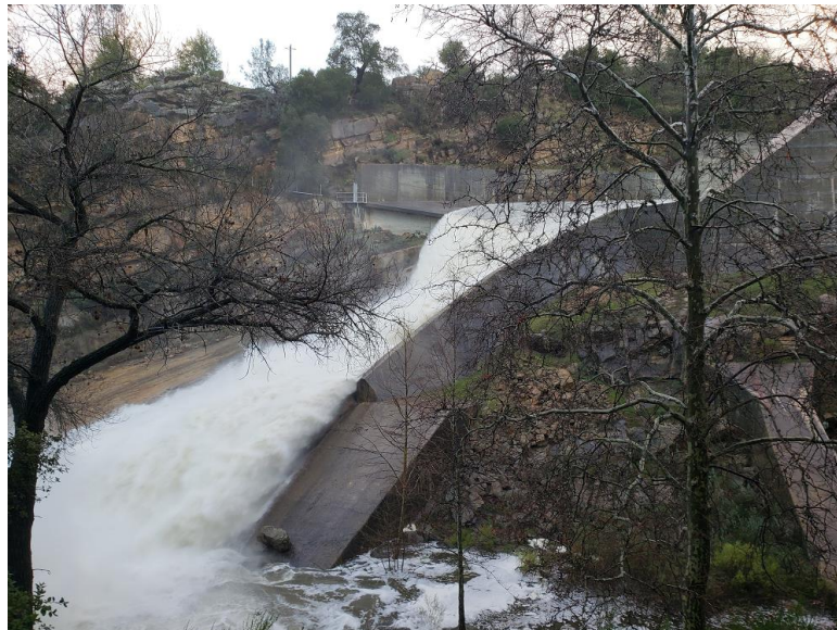
Salinas Dam spillway, February 2019.
