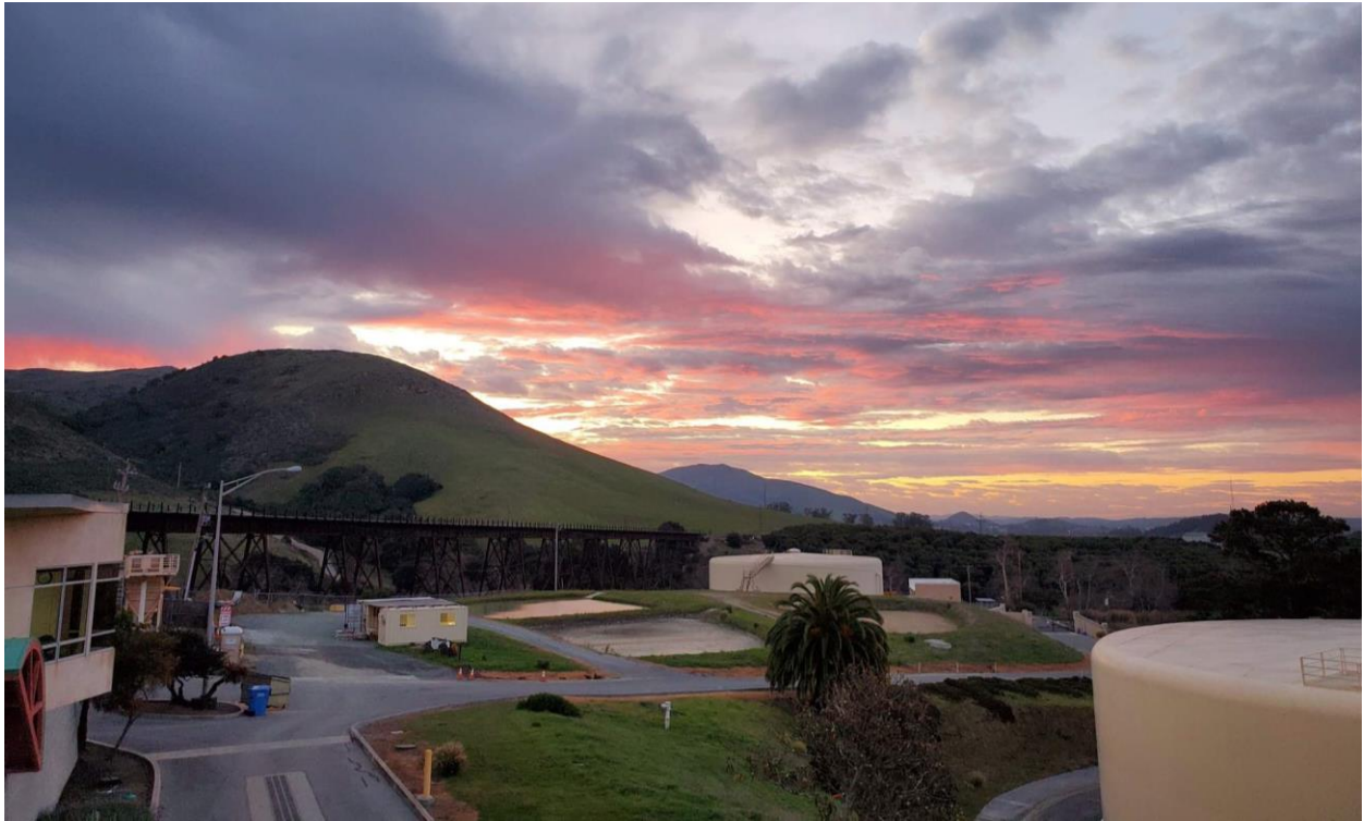
Stenner Canyon Water Treatment Plant.
