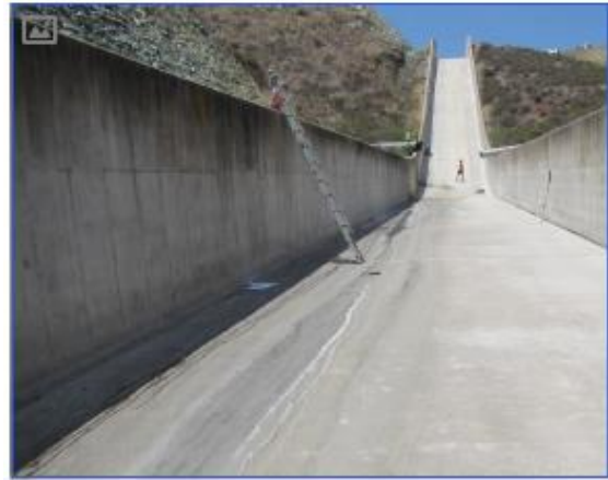
Whale Rock Dam Spillway.
