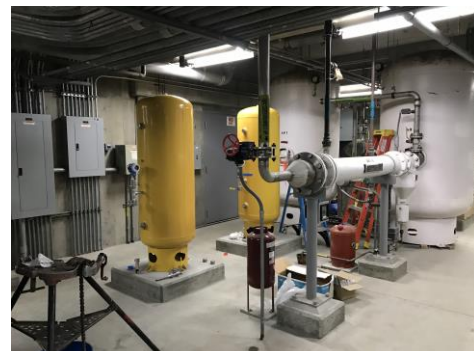
Installation of new Dilution Air Dryers.
