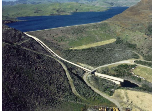
Whale Rock Reservoir Spillway
