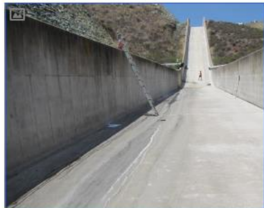
Whale Rock Dam Spillway.
